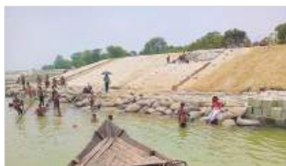
Revetment at Alatuli in Chapainawabganj Sadar upazila
