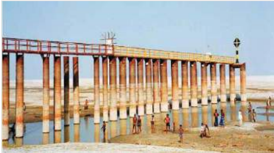
Figure 4.6: Permeable Groyne at Kamarjani of Jamuna River
