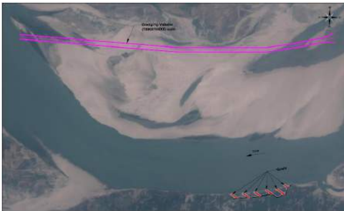
Figure 3.8: Kalihati Site with Dredging
