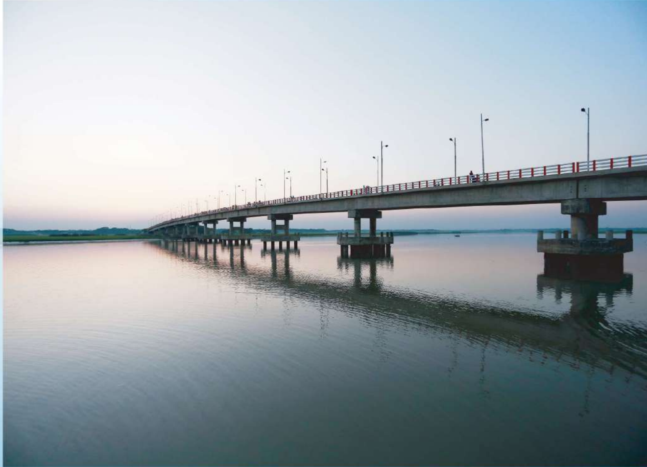
Baghmara Bridge, Bhola Sadar
