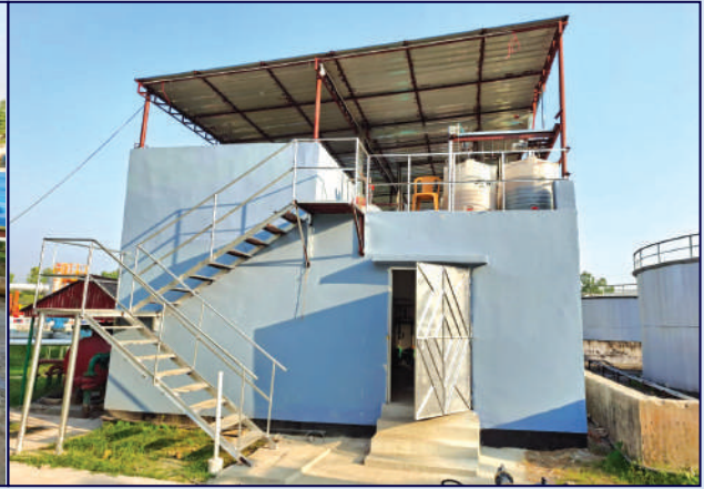
ETP installed for environment-friendly drainage of the produced water from wells at Bakhrabad field.
