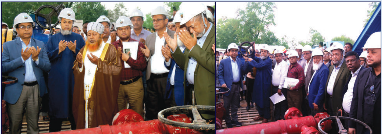
Mr. Md. Rezanur Rahman, Chairman, Petrobangla inaugurated gas production from Habiganj-5 well on 03-12-2025, which added about 26 MMCF gas daily in the national grid after workover.
