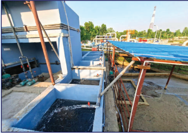
ETP installed for environment-friendly drainage of the produced water from wells at Bakhrabad field.
