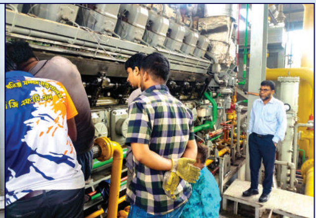
Maintenance activities of post 16000 operating-hours have been conducted by BGFCL's own manpower under the supervision of 02 experts of EGS, Romania, an authorized agency of manufacturer.
