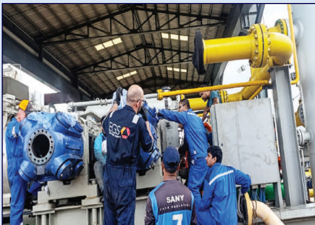
Maintenance activities of post 16000 operating-hours have been conducted by BGFCL's own manpower under the supervision of 02 experts of EGS, Romania, an authorized agency of manufacturer.
