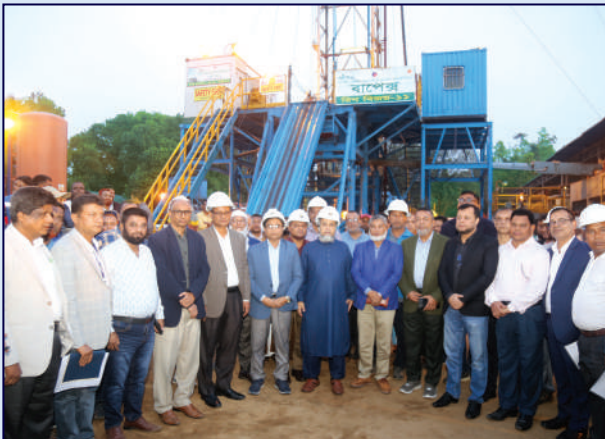
Successful completion of workover of Habiganj-5 well, paving the way for nearly an additional 26 MMscfd gas supply to the national grid.
