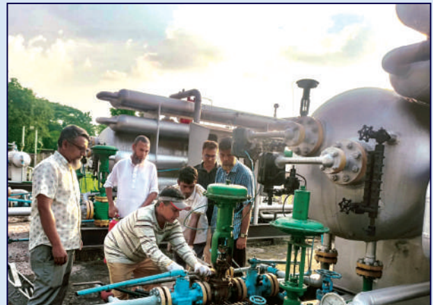
PCV maintenance work at Meghna Gas Field.
