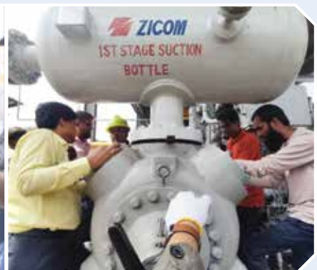
Replacement of PCV of Process Plant 3 at Habiganj Gas Field.
