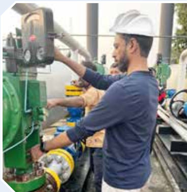
Maintenance work for the PCV of gas process plant at Titas Gas Field.
