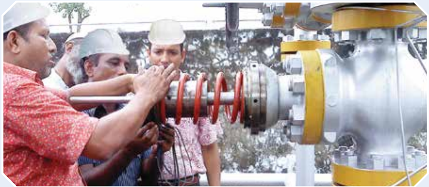
Maintenance work for the PCV of gas process plant at Titas Gas Field.
