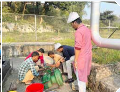
Replacement of PCV of Process Plant 3 at Habiganj Gas Field.
