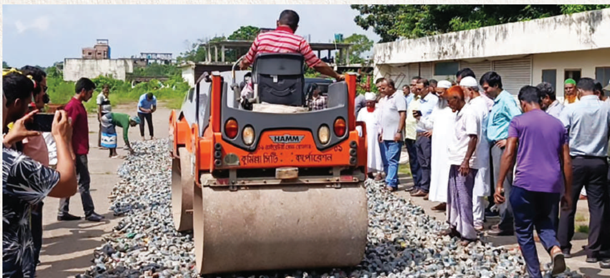
Destroying regulators removed during illegal disconnections
