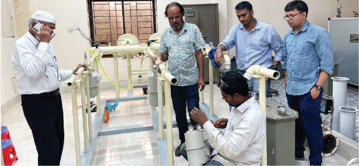
Commissioning of Testing and commissioning of Diaphragm Meter Testing Bench.
