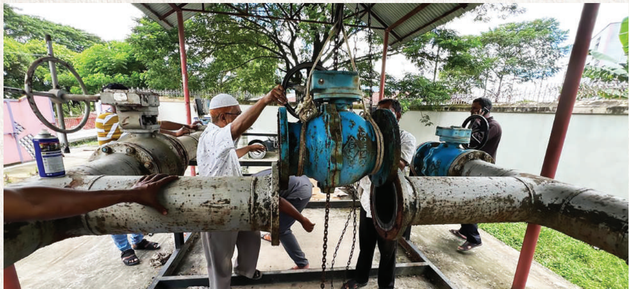
8 inch valve replacing work at Cumilla EPZ DRS
