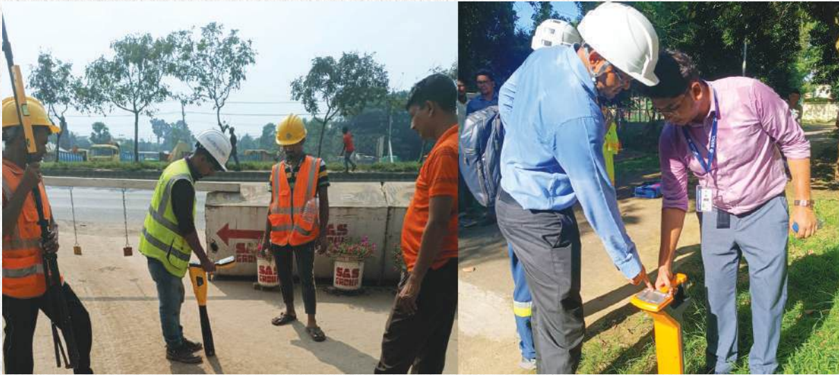
Hands on works for pipeline detecting to prepare GIS mapping
