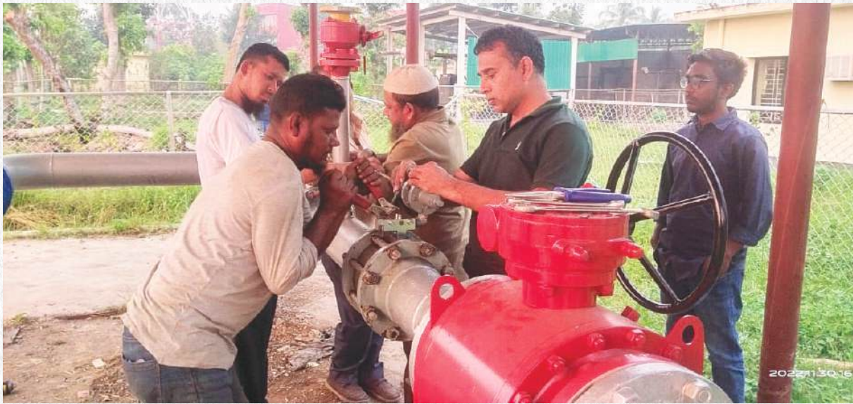
Emergency maintenance and repair work of Debidwar/BKB gas field TBS
