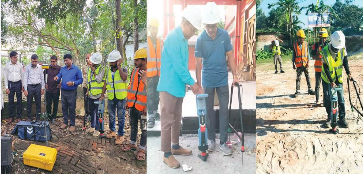
Coating defect survey work of pipeline in Cumilla area
