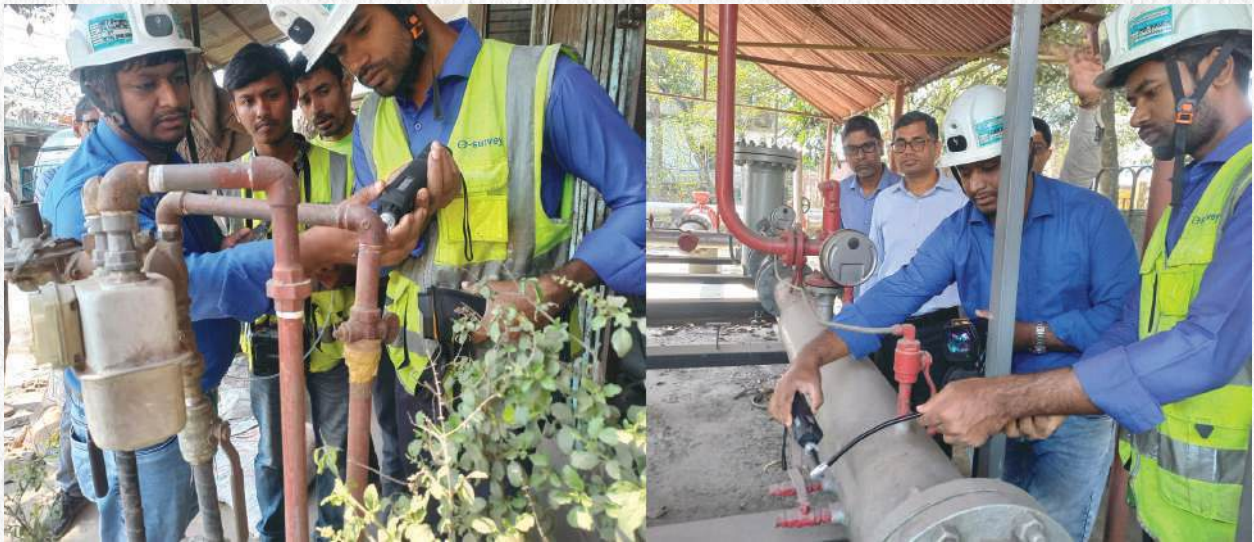
Leakage detection activities is going on with handy gas leakage detector
