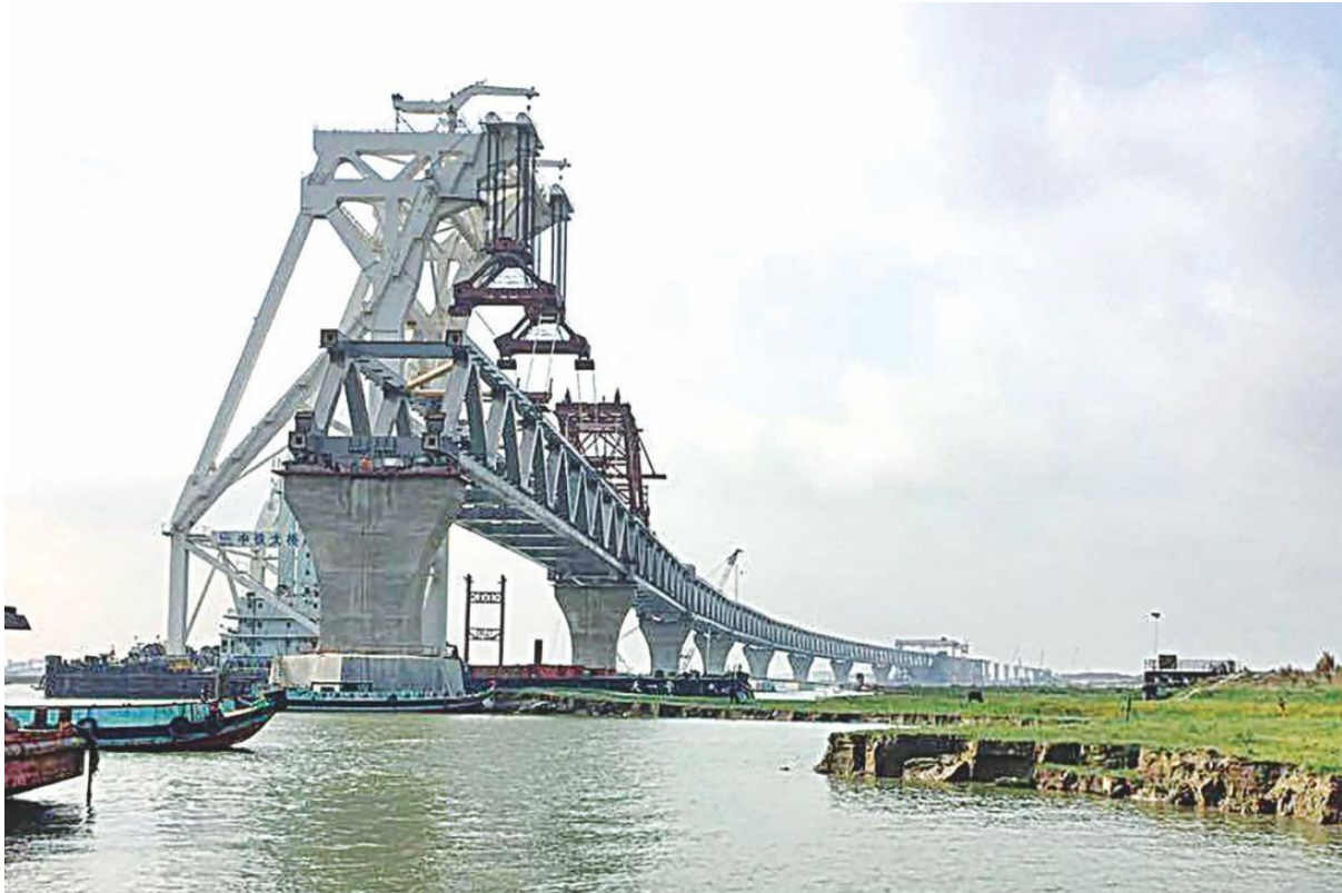
Padma Bridge under construction
