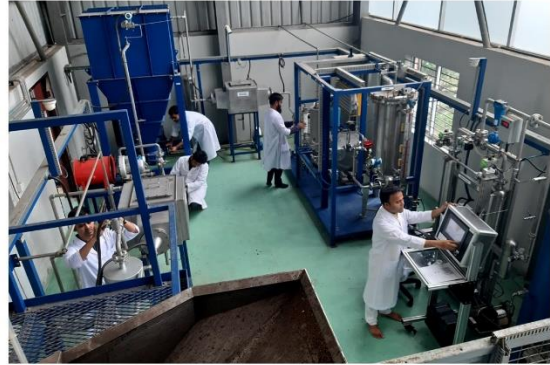
Biomass Gasification Derived Hydrogen Production Plant
