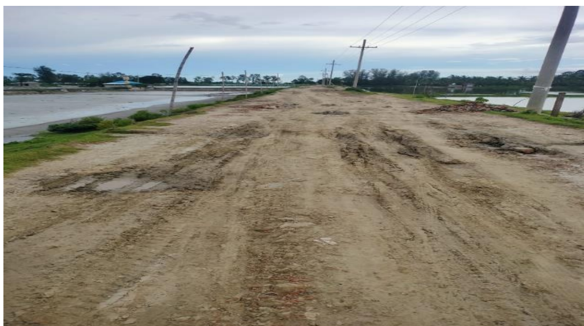
Photo 32: Physical verification of Road transportation infrastructure in rural areas of Bangladesh
