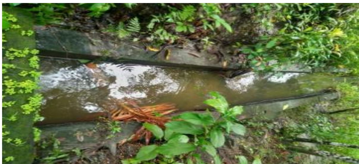
Photo 29: Physical verification of the drainage system
