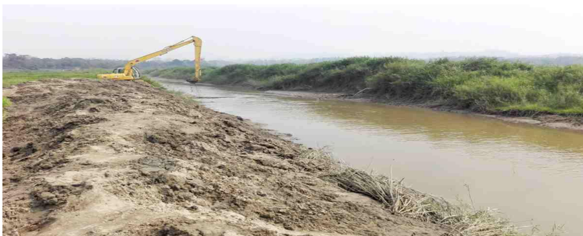
Photo 14 : canal re/excavation
