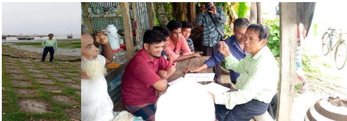
Physical observation of Meghna riverbank protective work by Consultant at Noakhali
