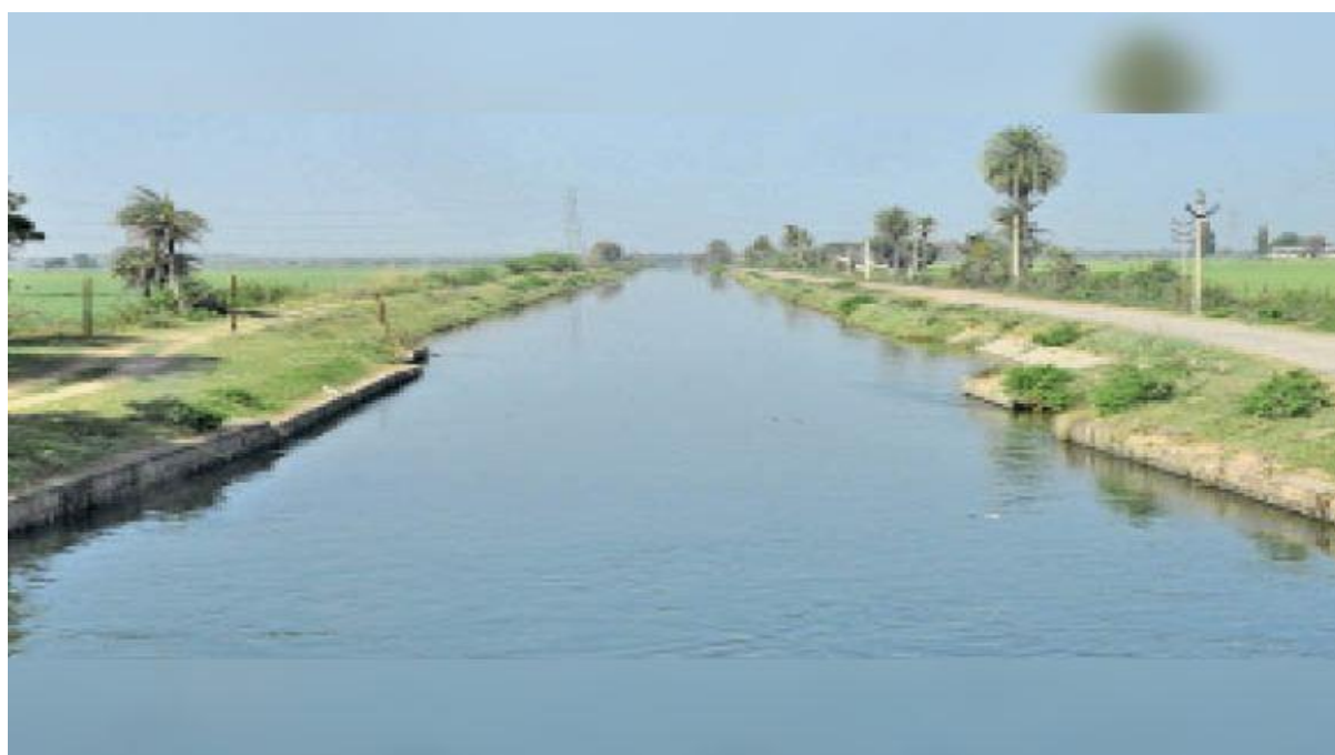
Photo 31: canal excavation and re-excavation for navigation improvement and irrigation purposes
