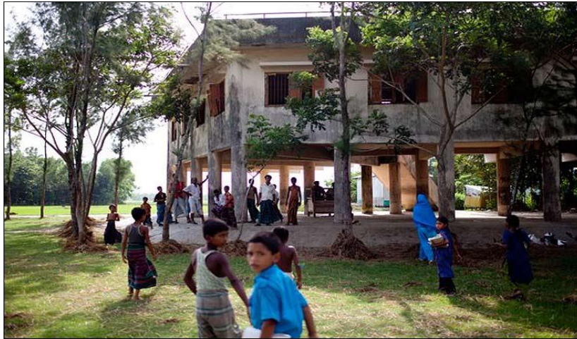
Photo 11: school cum cyclone shelters
