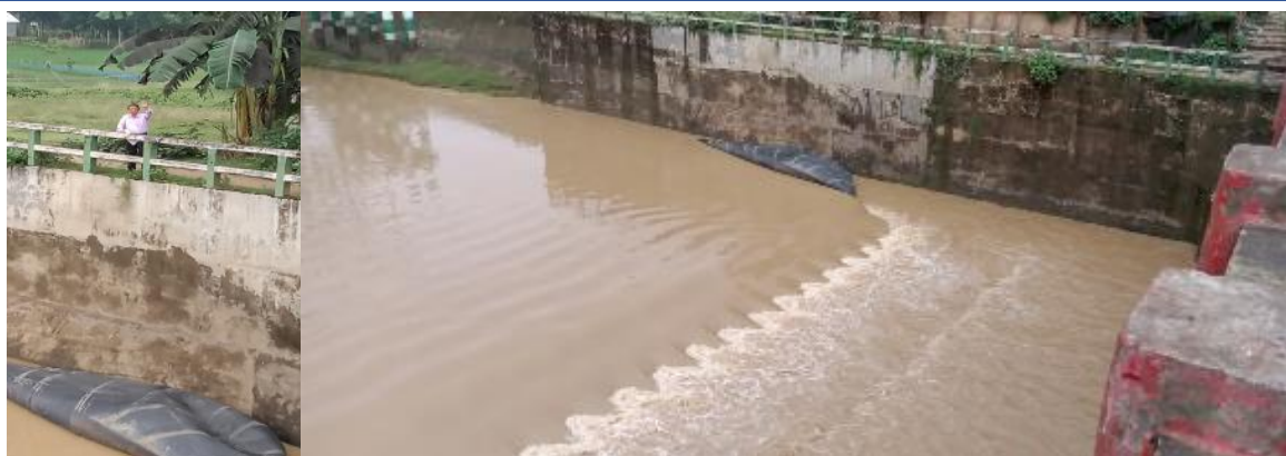
Physical observation of Chellakhali river rubber dam irrigation project by Consultant in Sherpur
