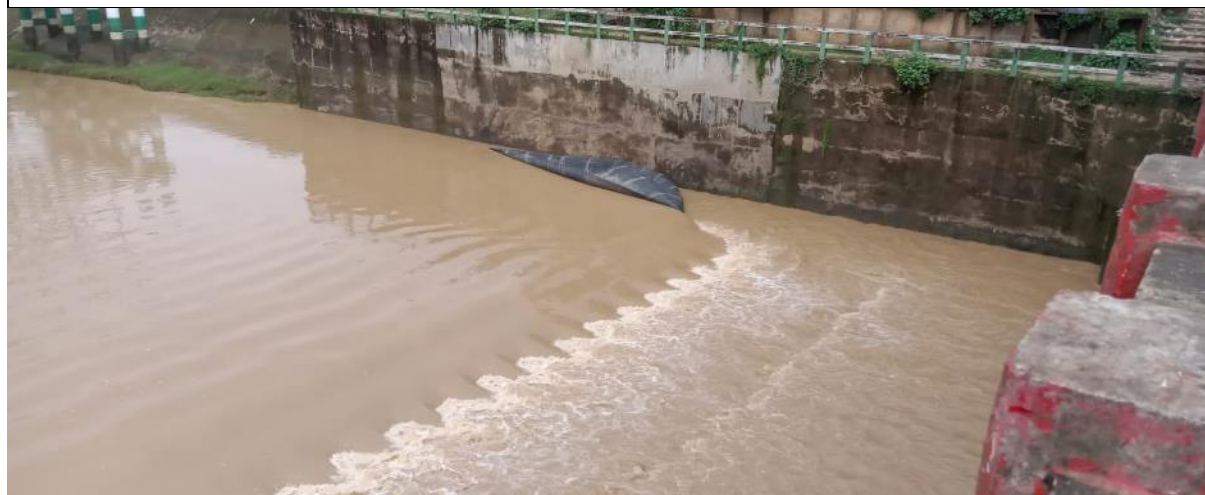
Photo 24: Rubber Dam Irrigation Project in Chellakhali River in Nalitabari Upazila of Sherpur district.
