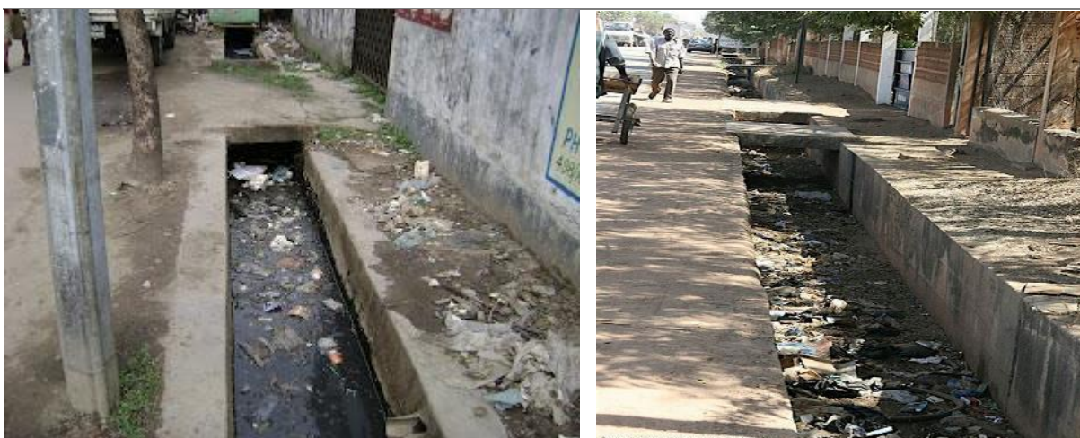
Photo 9 : Pictures – urban drainage system for removing logged and wastewater
