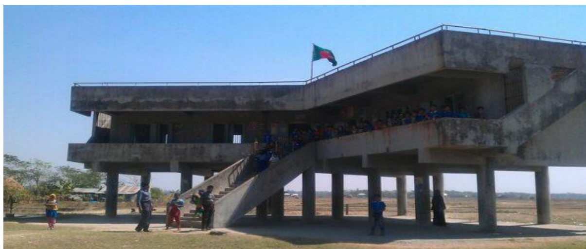
Photo 30: physical verification of school cum cyclone shelter in coastal Bangladesh
