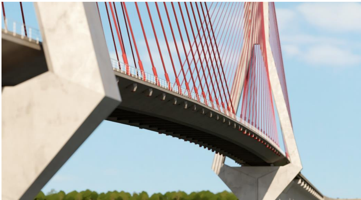
Figure 7. Cable Stayed bridge at Matlab Uttar-Gazaria. View from riverbank.
