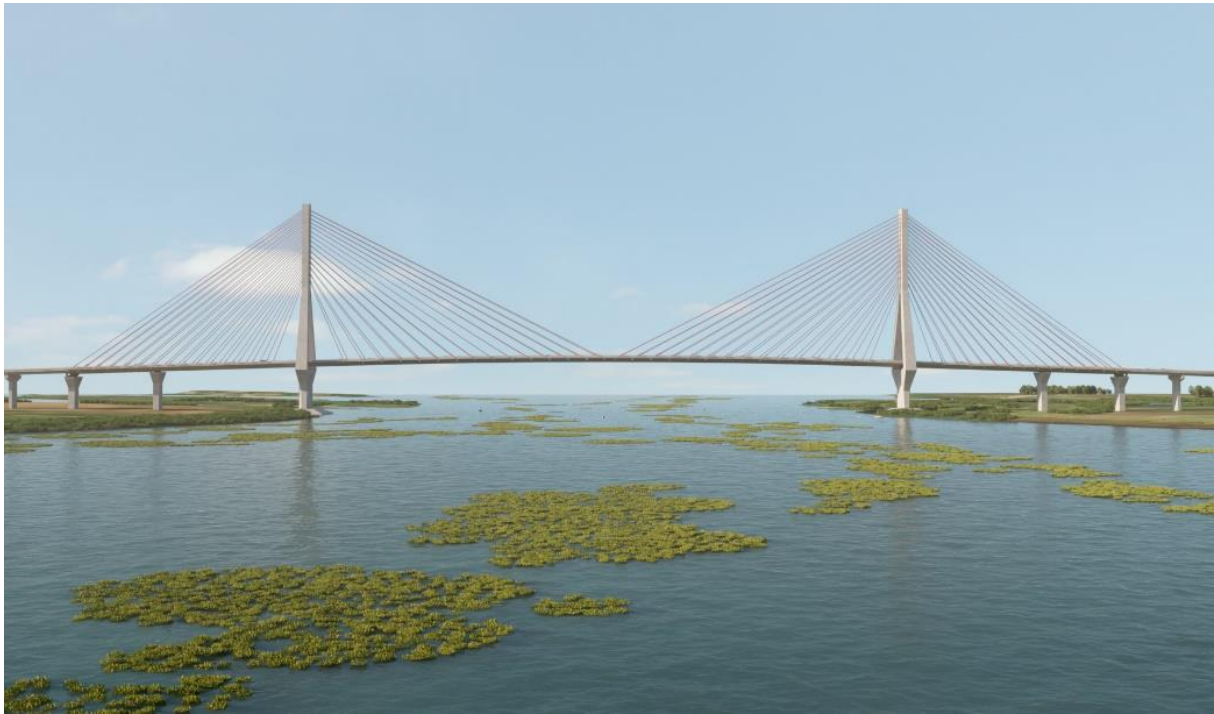
Figure 8. Cable Stayed bridges at Matlab Uttar-Gazaria. General view
