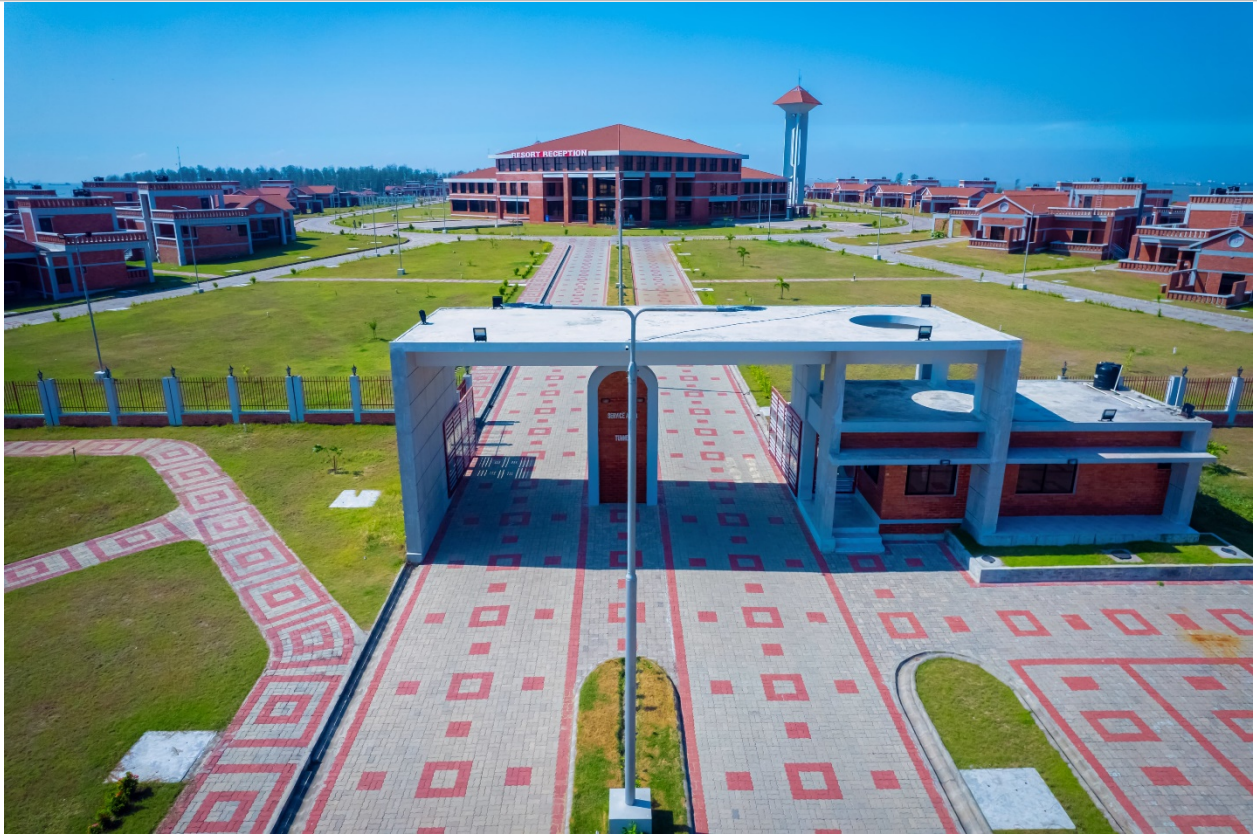
Gate House, Internal Roads & Walkway
