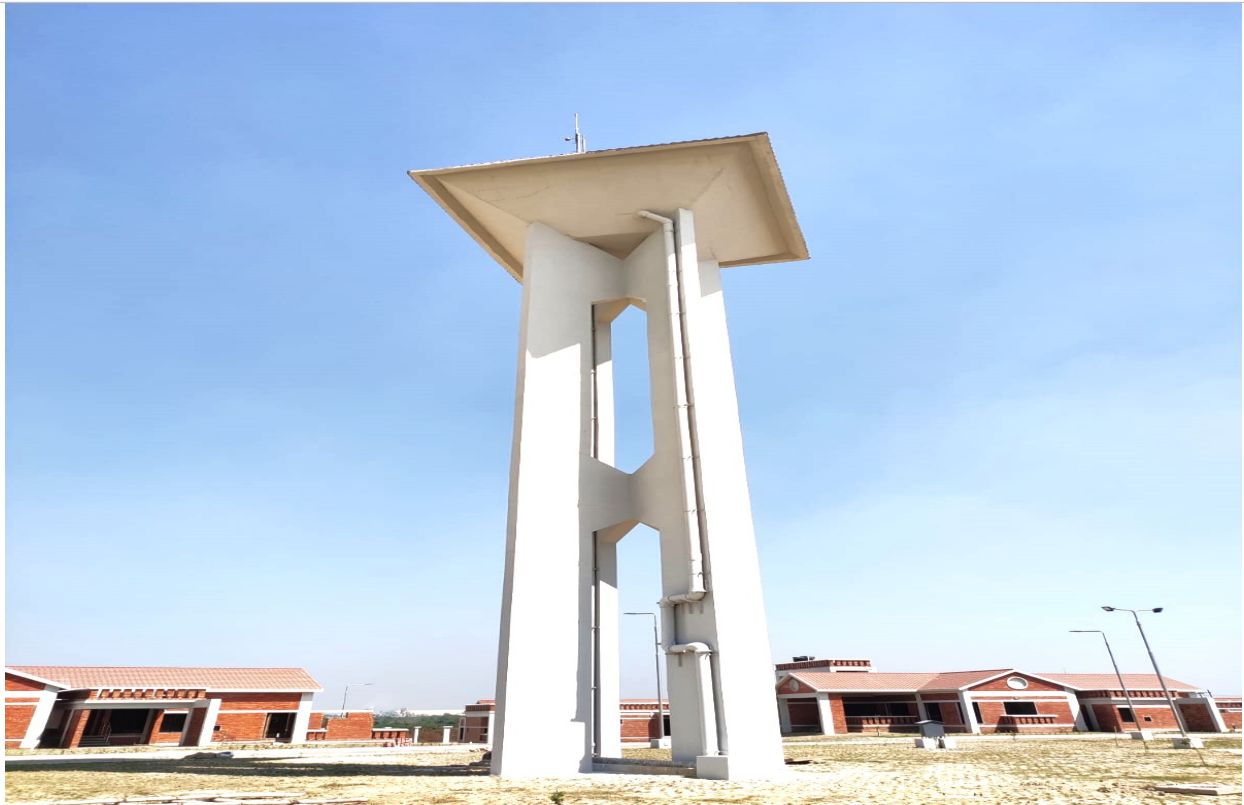
Over Head Water Tank
