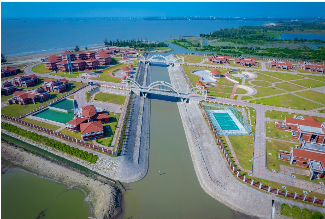
Bridges over canal, Slope Protection & Boundary Wall
