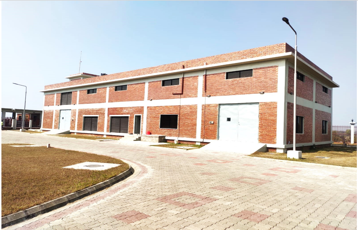
Sub-Station & Generator Building
