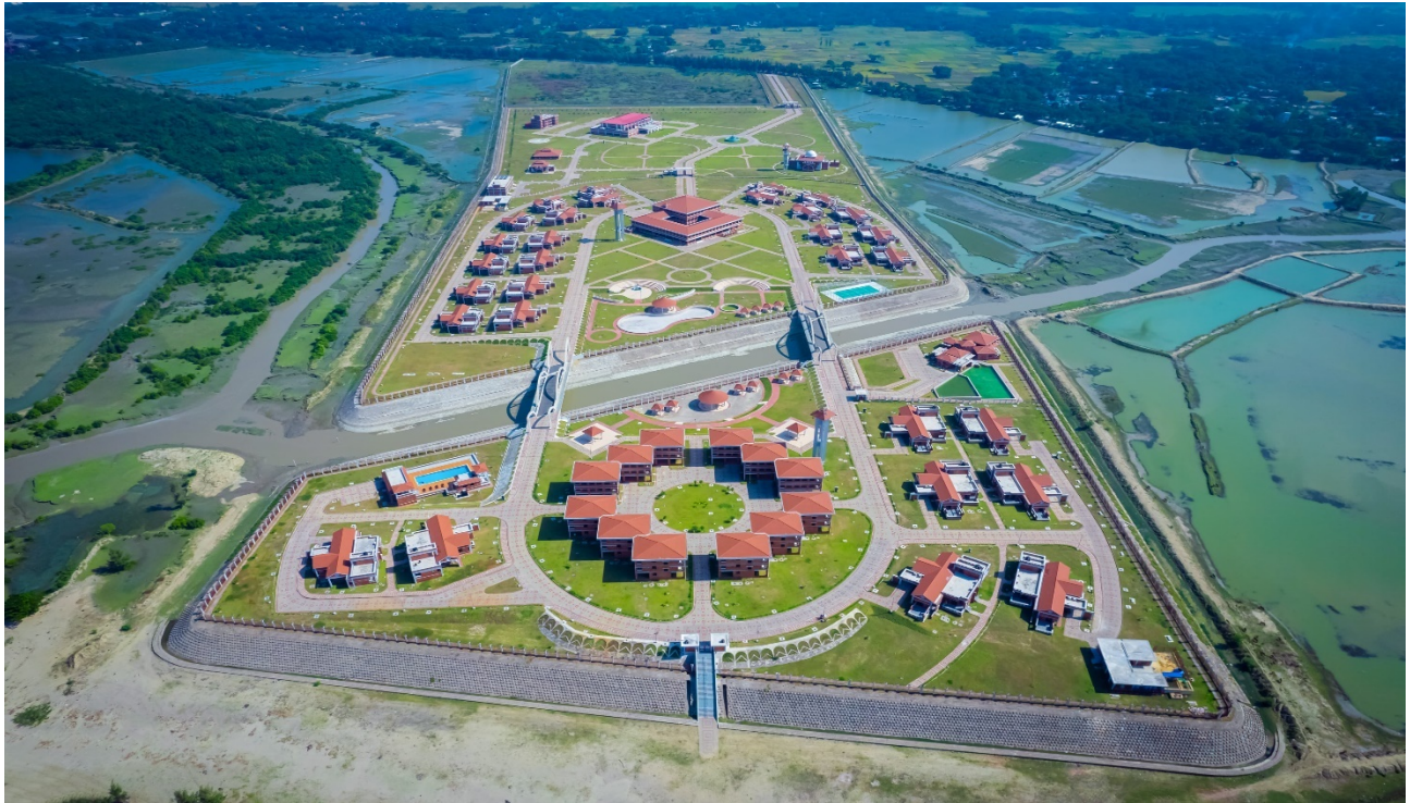
Topographical View of Service Area Facilities, Bangladesh Bridge Authority at Chattogram
