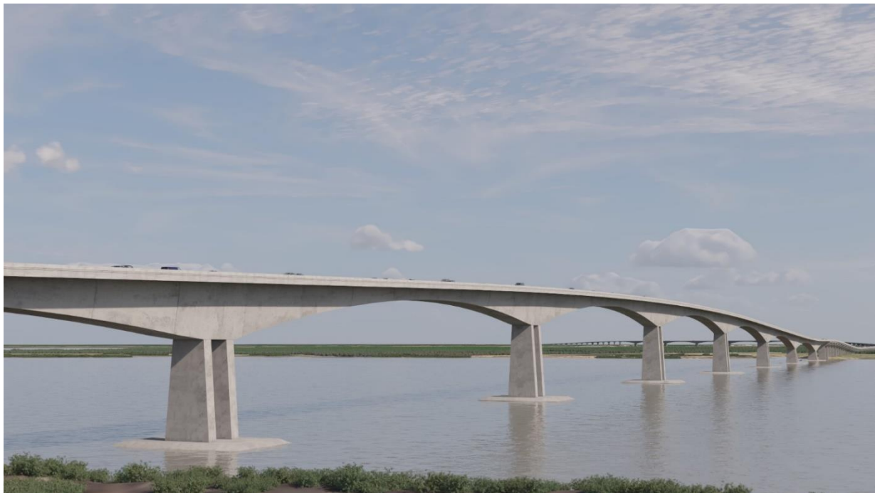
Figure 14 Image of balanced cantilever spans proposed for Barishal-Bhola.
