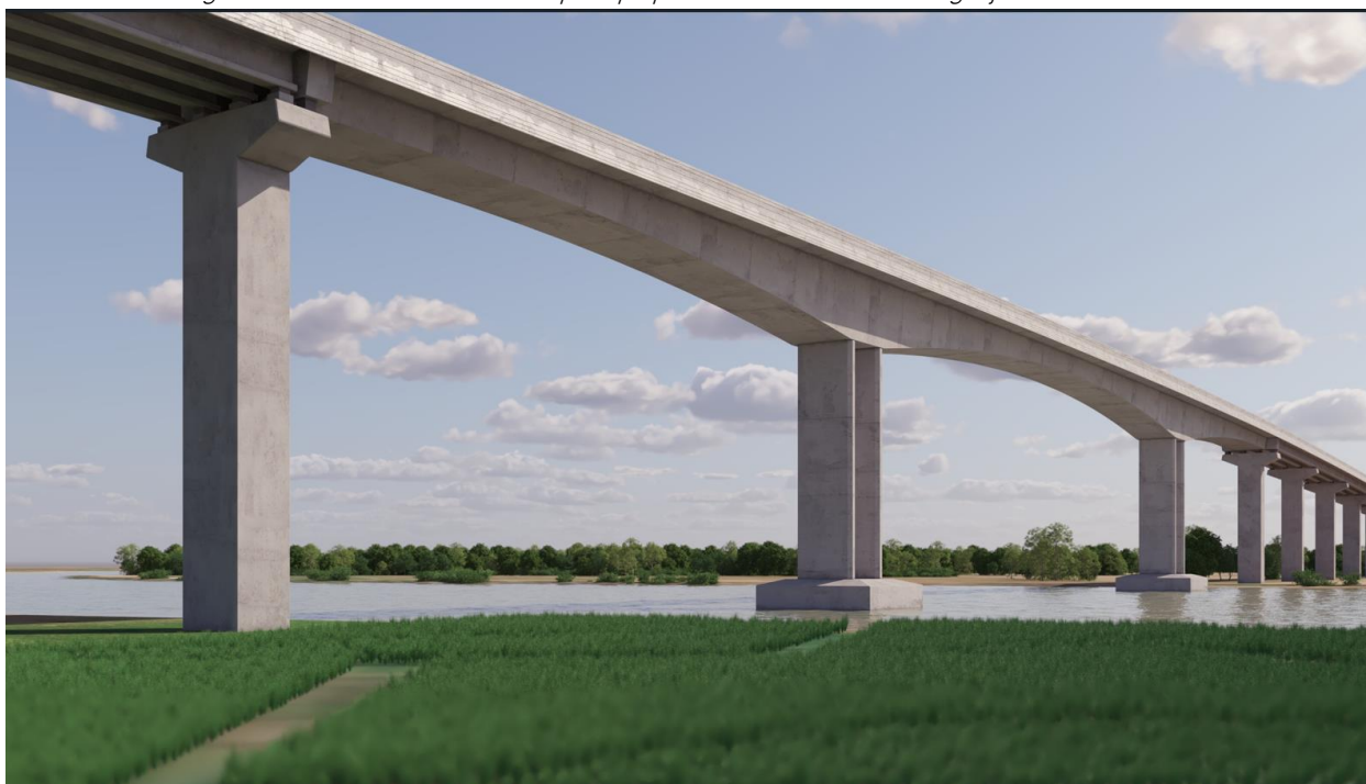
Figure 26 Balanced Cantilever Bridge proposed for channels in Netrokona-Sunamganj.
