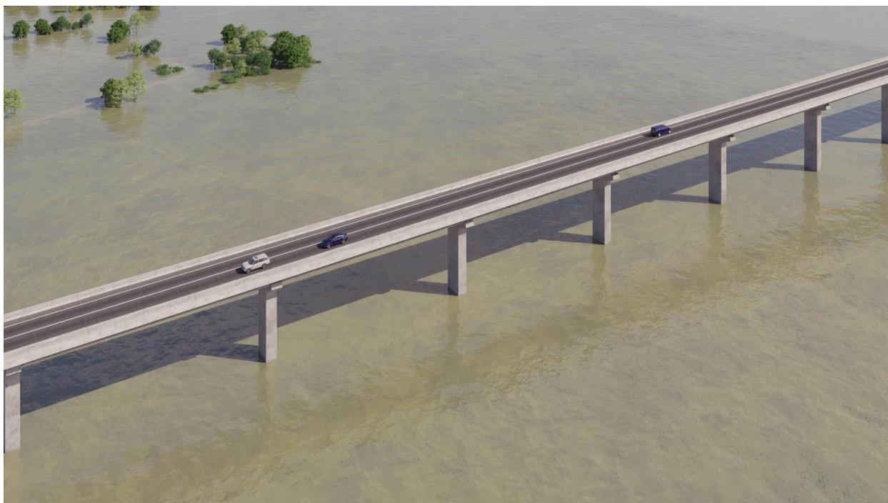
Figure 25 Flooded Precast I-Girder Spans proposed for Netrokona-Sunamganj elevated road.
