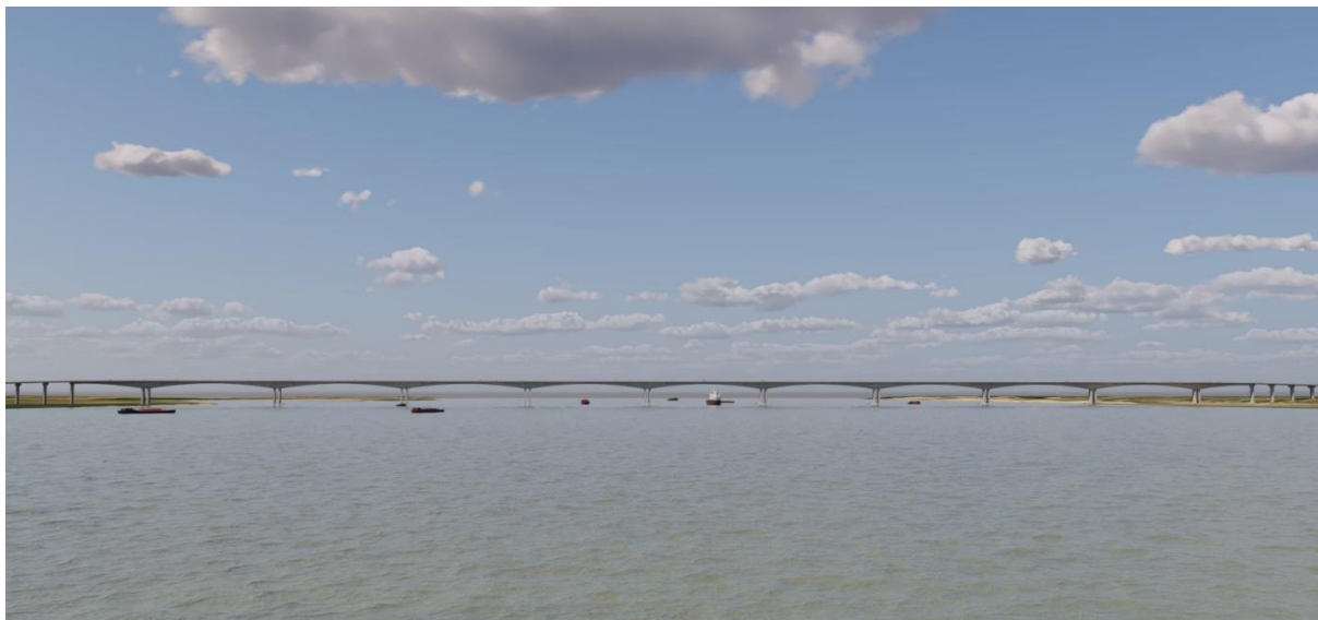
Figure 25. Balanced cantilever spans proposed.
