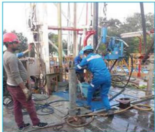
Workover activities of Rashidpur-5
