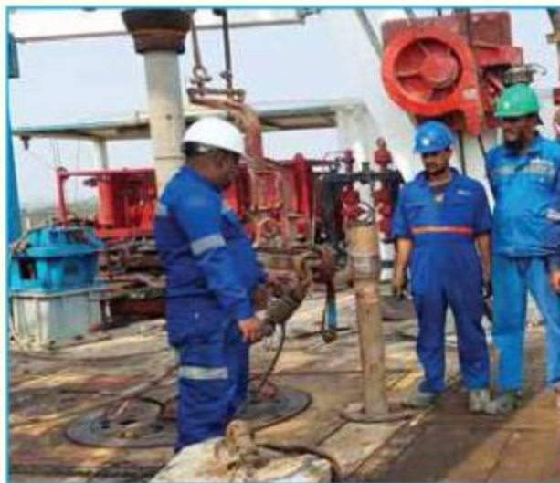
Workover activities of Kailastila-2
