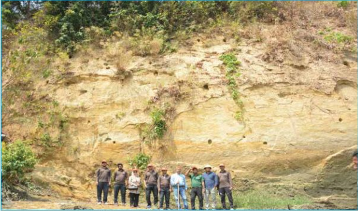
Geological Survey along Karnaphuli River of Patiya Structure
