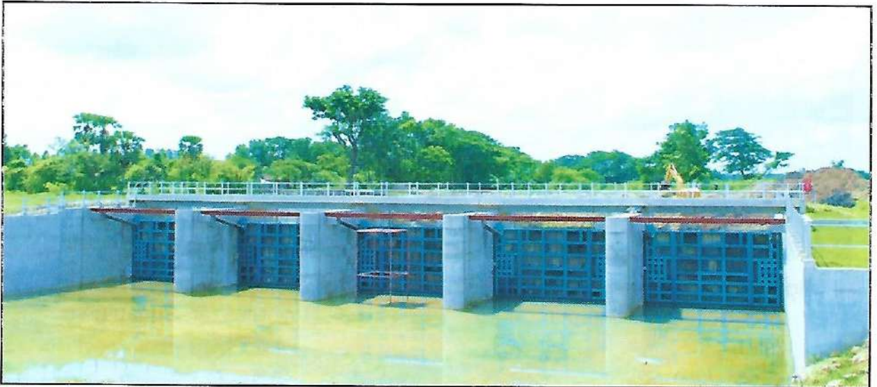
Figure 18: Hydraulic Elevated Dam at Anowara, Chottogram.
