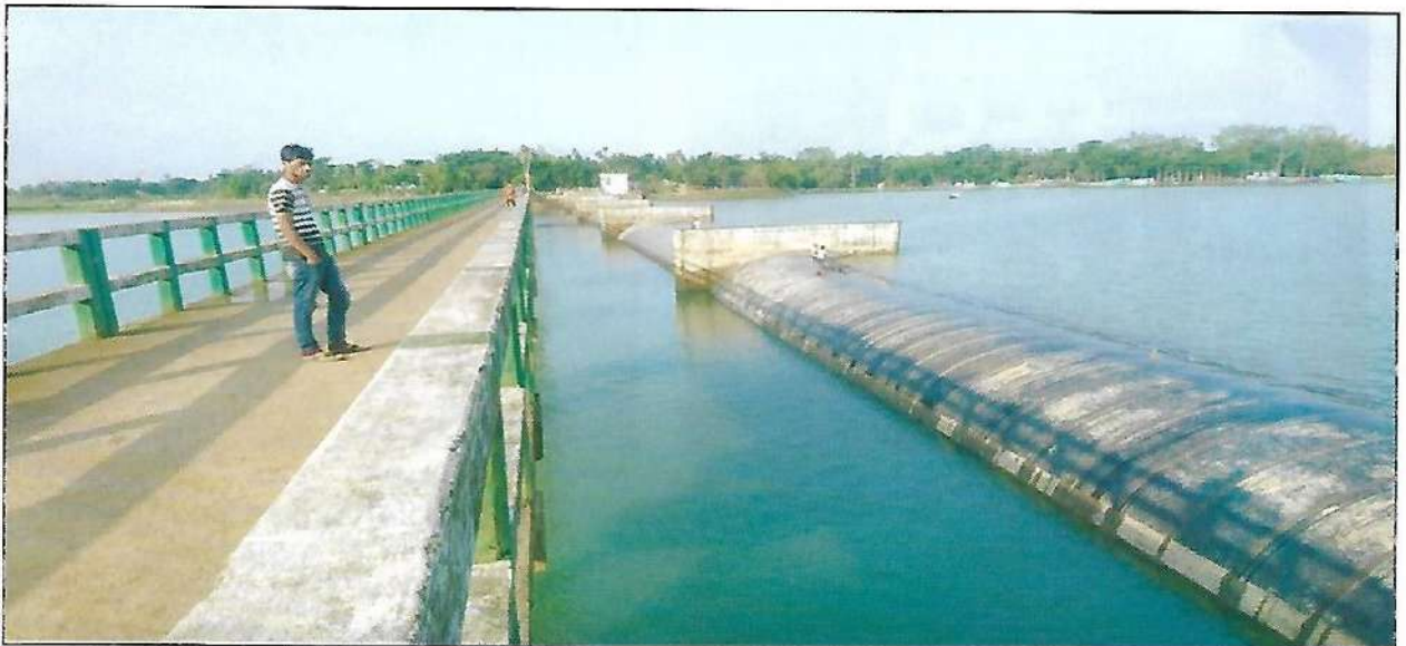
Figure 19: Michhakhali Rubber Dam, Bishambharpur, Sunamganj.
