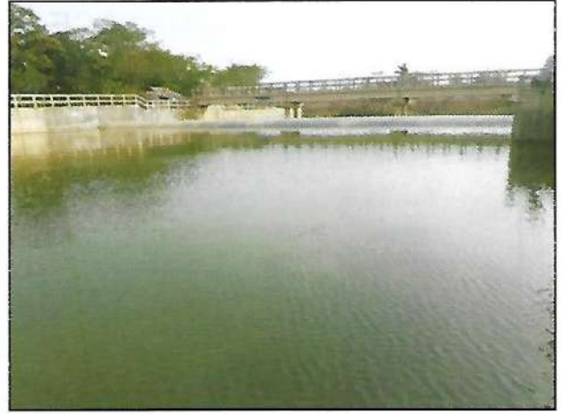
Figure 22: Chilai River Rubber Dam, Doyarabazar, Sunamganj.
