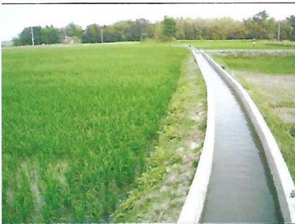
Figure 25: RCC Channel at Habiganj
