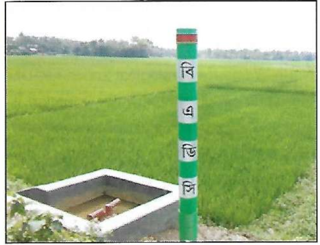
Figure 6: Electrically Operated Deep Tube Well and Buried Pipe Line.
