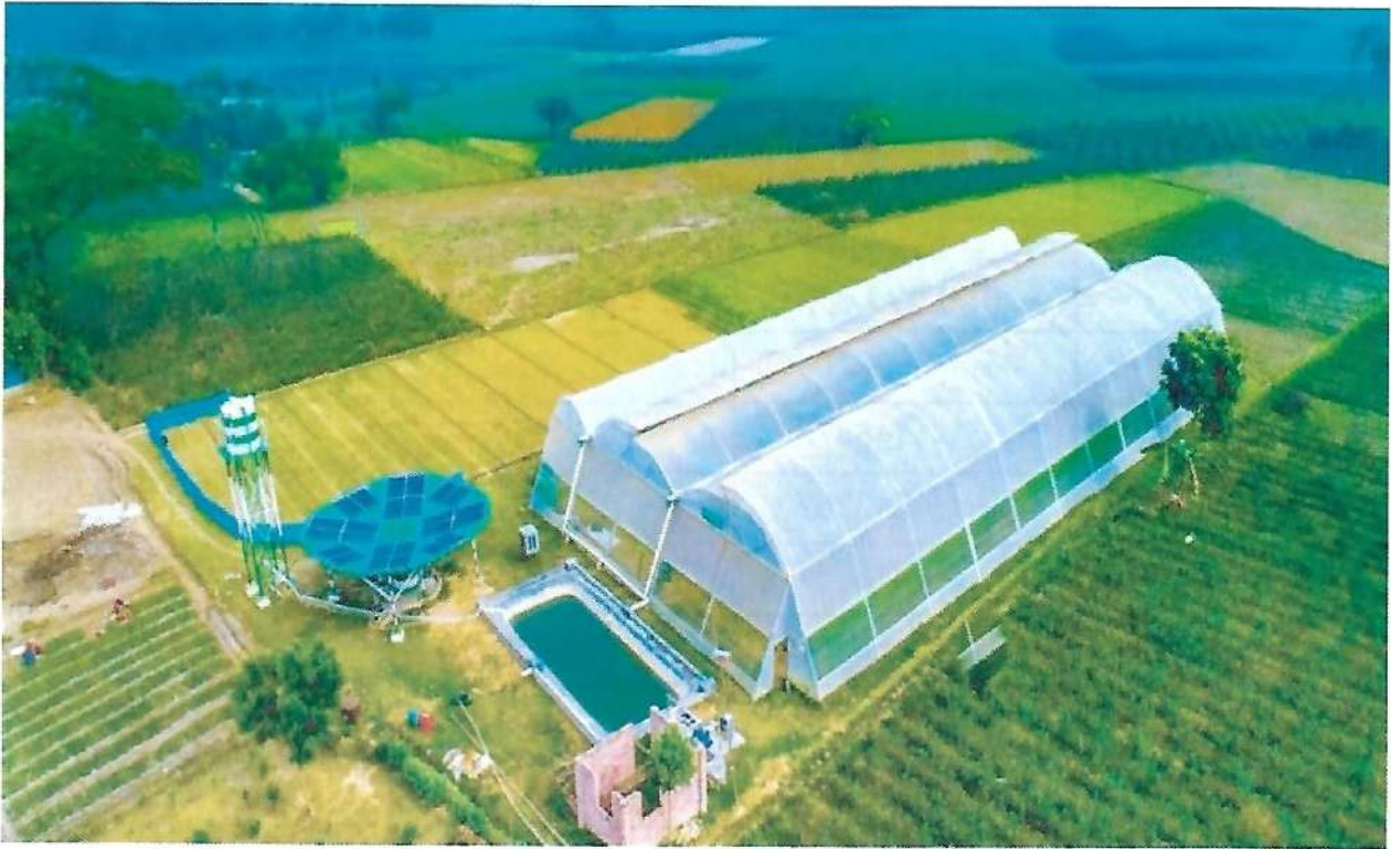
Figure 10: Solar Energized Dug Well, Panisara Village, Jhikargacha, Jessore.
