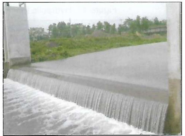
Figure 24: Submerged Weir, B. Baria.
