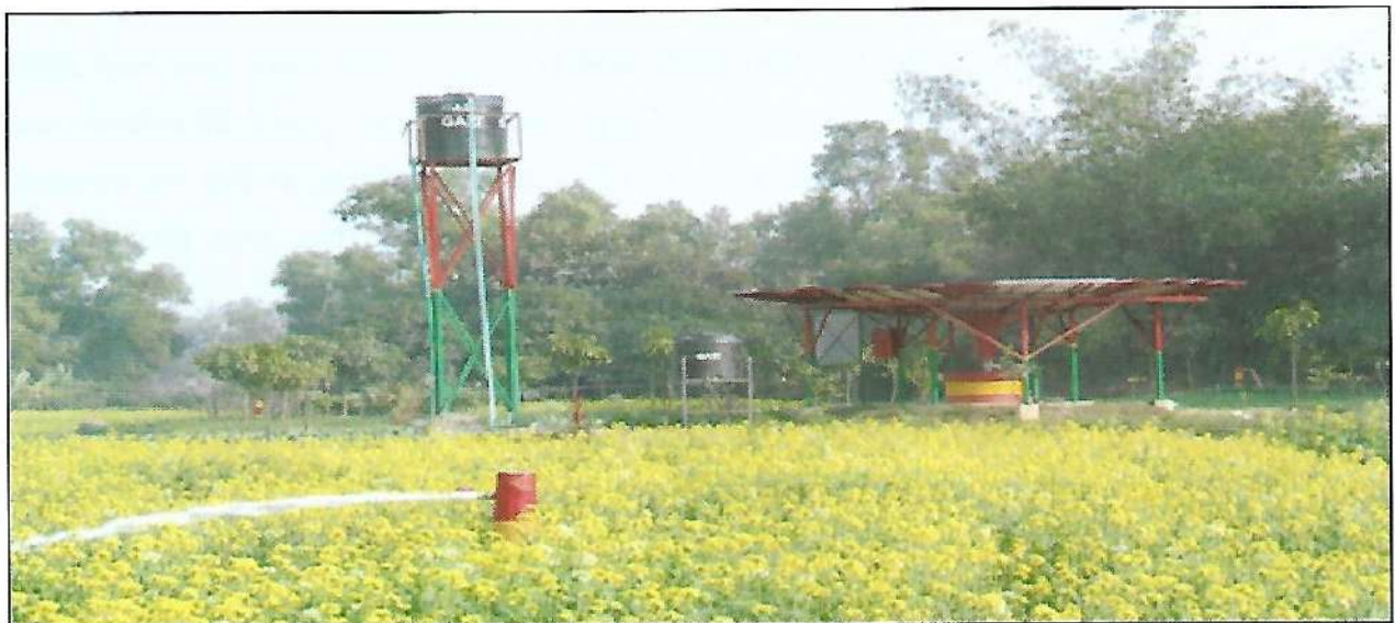
Figure 9: BMDA Solar Energized Dug Well in Shapahar Upazila, Naogaon.
