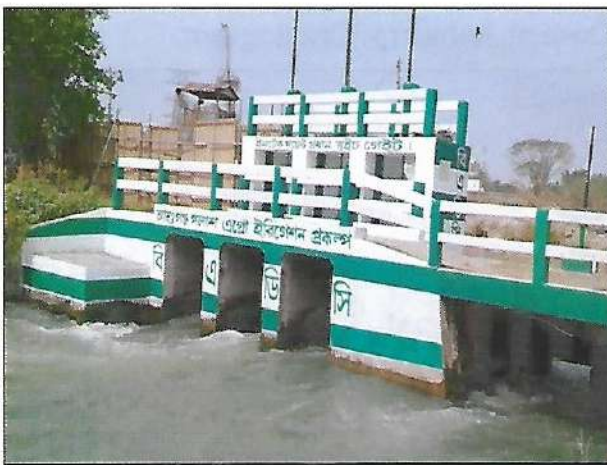
Figure 23: Intake Point of Sluice Gate, B. Baria.
