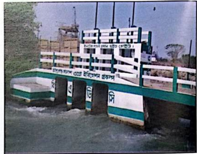
Figure 23: Intake Point Sluice Gate, B. Baria
