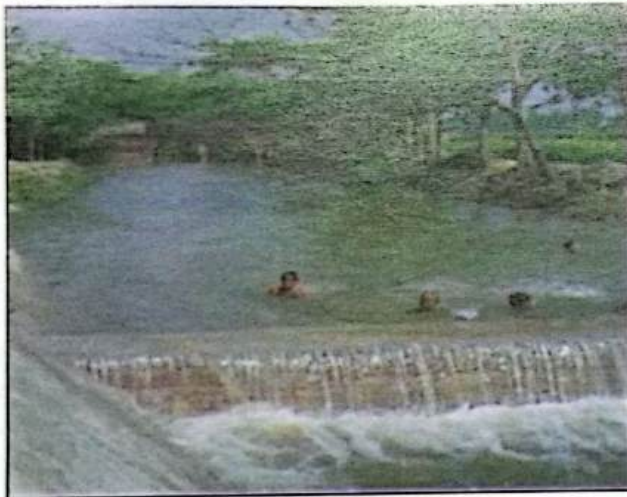
Figure 22: Submerged Weir, B. Baria
