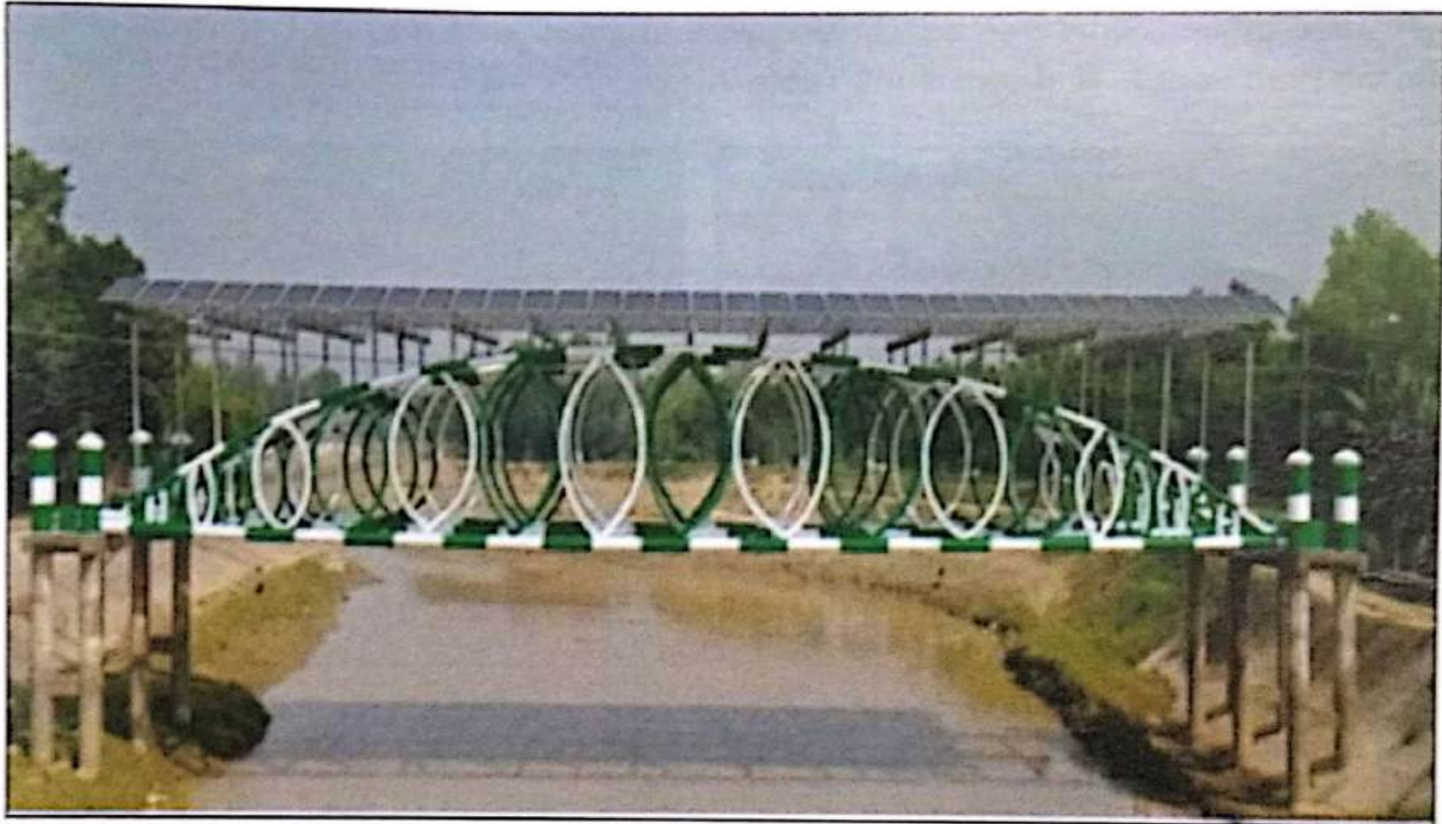
Figure 26: 5-cusec solar pump-Nalitabari-Sherpur
