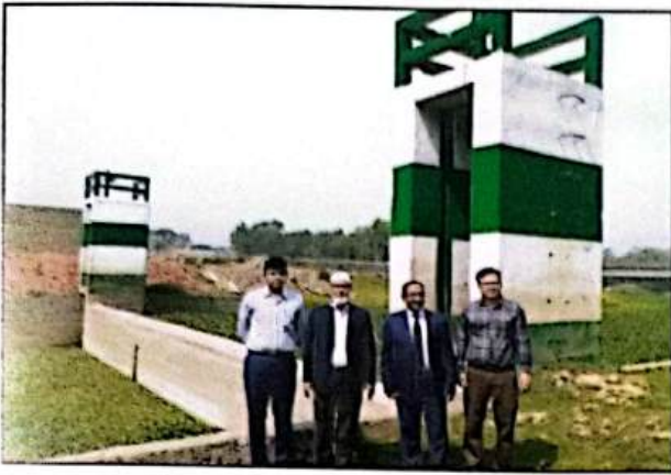
Figure 14: Submerged Weir, B. Baria
