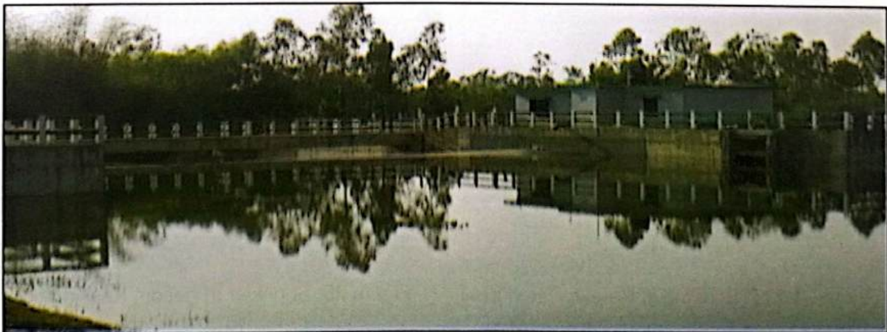
Figure 20: Sorai Khal Rubber Dam, Lohagara, Chattogram
