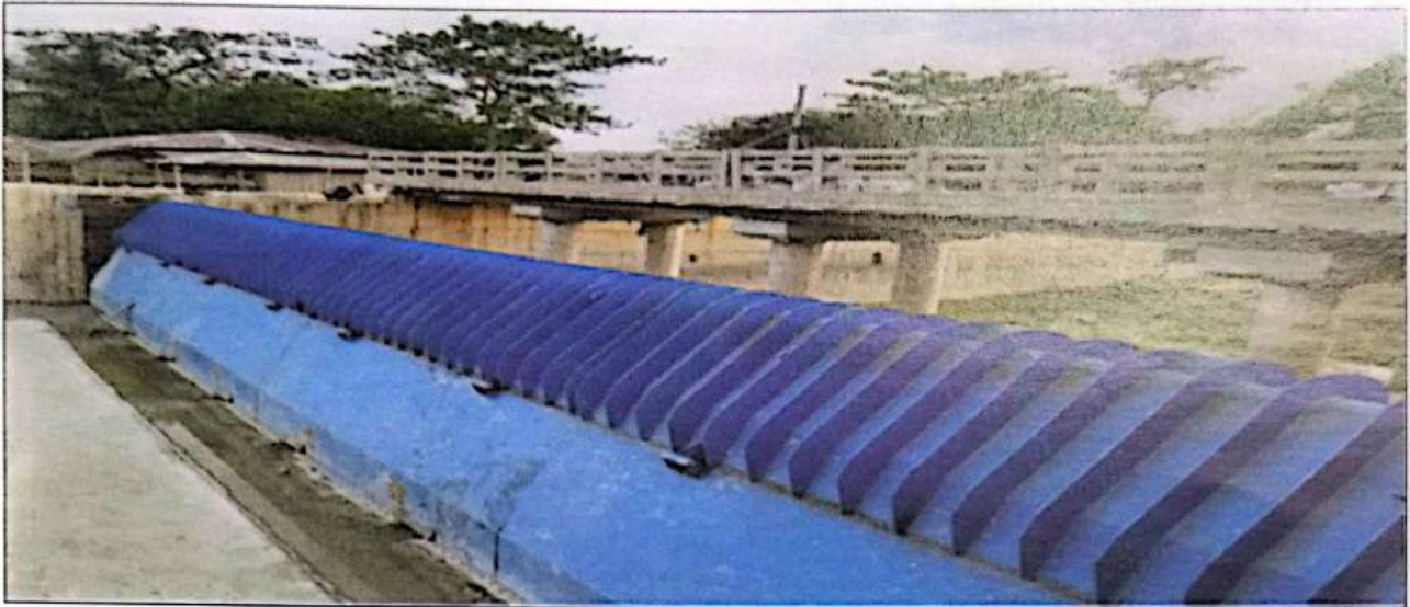
Figure 18: Harbang Hydraulic Elevator Dam, Chakaria, Cox'sbazar
