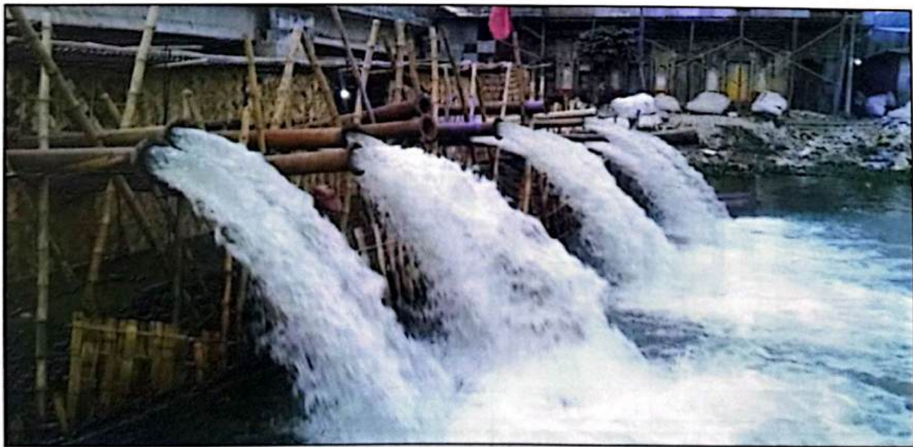
Figure 32: Floating pump, Boaljhuri, Haziganj, Chadpur
