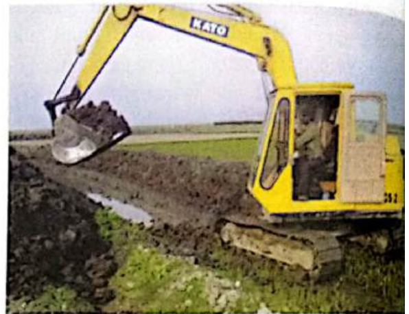
Figure 31: Re-excavation of Khal at Kishoreganj
