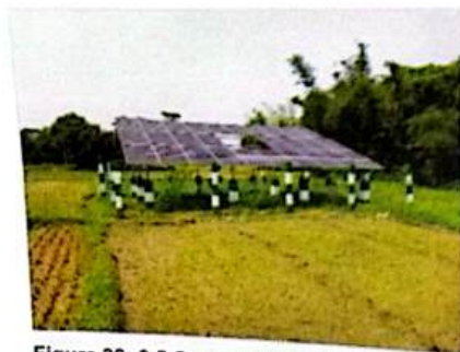
Figure 38: 0.5 Cusec Solar LLP at Brahmanpara Upazila, Cumilla
