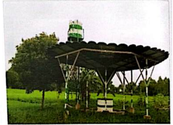
Figure 22: BADC Solar operated Dug well at Chhagalnaiya Upazila, Feni.
