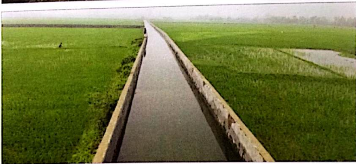
Figure 49: Gravity flow irrigation at Ashuganj-Polash agro-irrigation project by BADC
