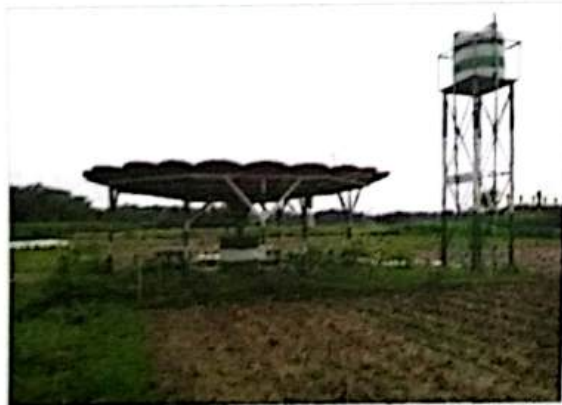
Figure 23: BADC Solar operated Dug well at Daulatpur, Kustia.
