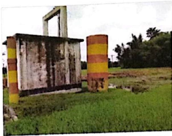
Figure 11: BMDA DTW at Naldanga Upazila, Nator
