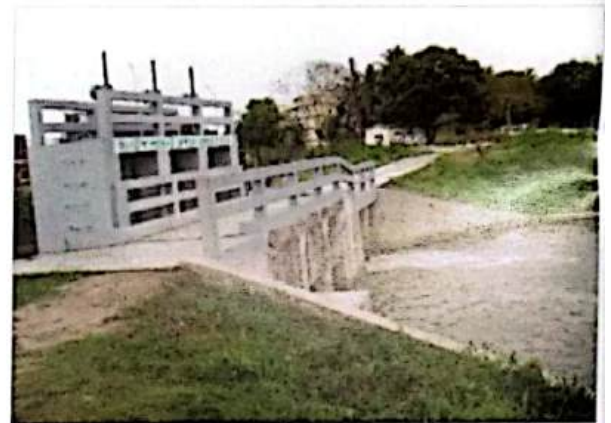
Figure 33: Intake point of Regulator at Ashuganj-Palash Agro Irrigation Project by BADC
