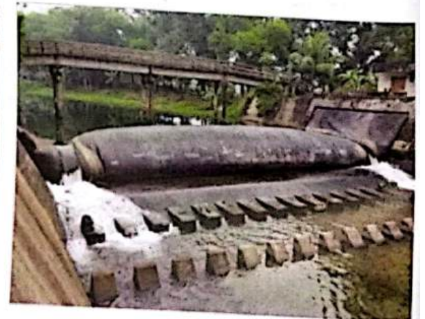
Figure 48: Mohamaya Rubber Dam at Mirsharai Upazila, Chattogram by BWDB.
