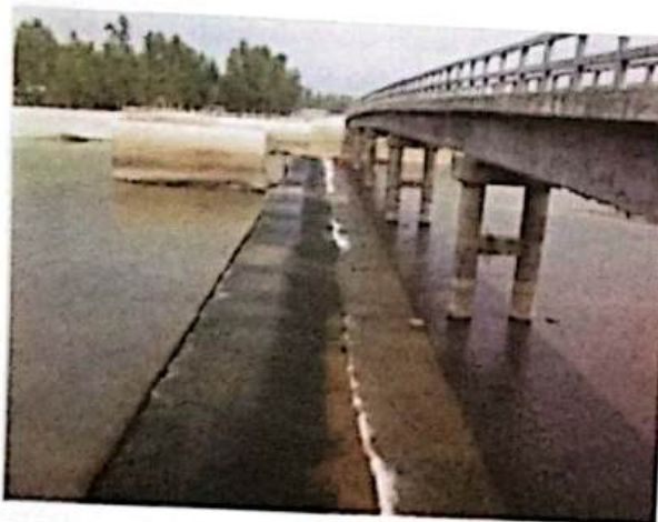
Figure 47: Zinziram Nodi Rubber Dam at Raumari upazila, Kurigram by LGED.
