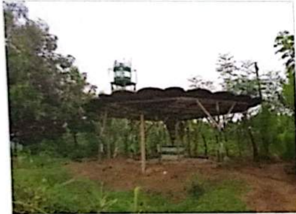
Figure 21: BADC Solar operated Dug well at Madhupur Upazila, Tangail
