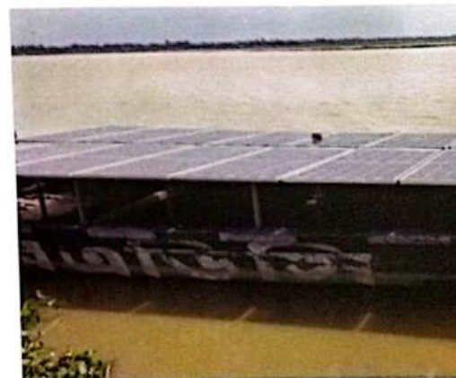
Figure 44: Boat Mounted Floating Solar LLP at T
