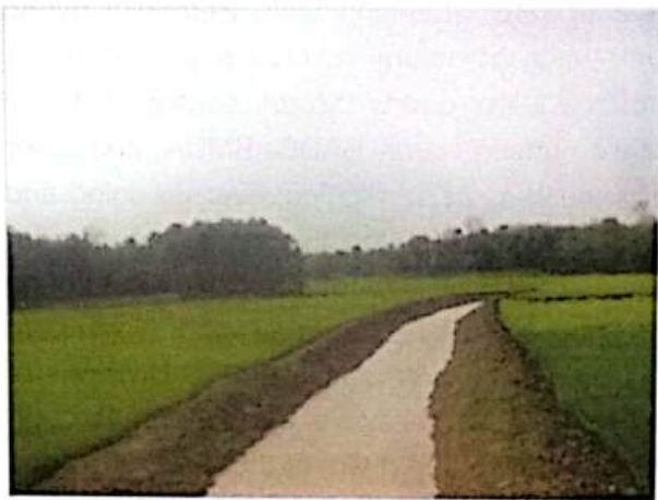
Figure 30: Re-excavated Khal at Narsingdi
