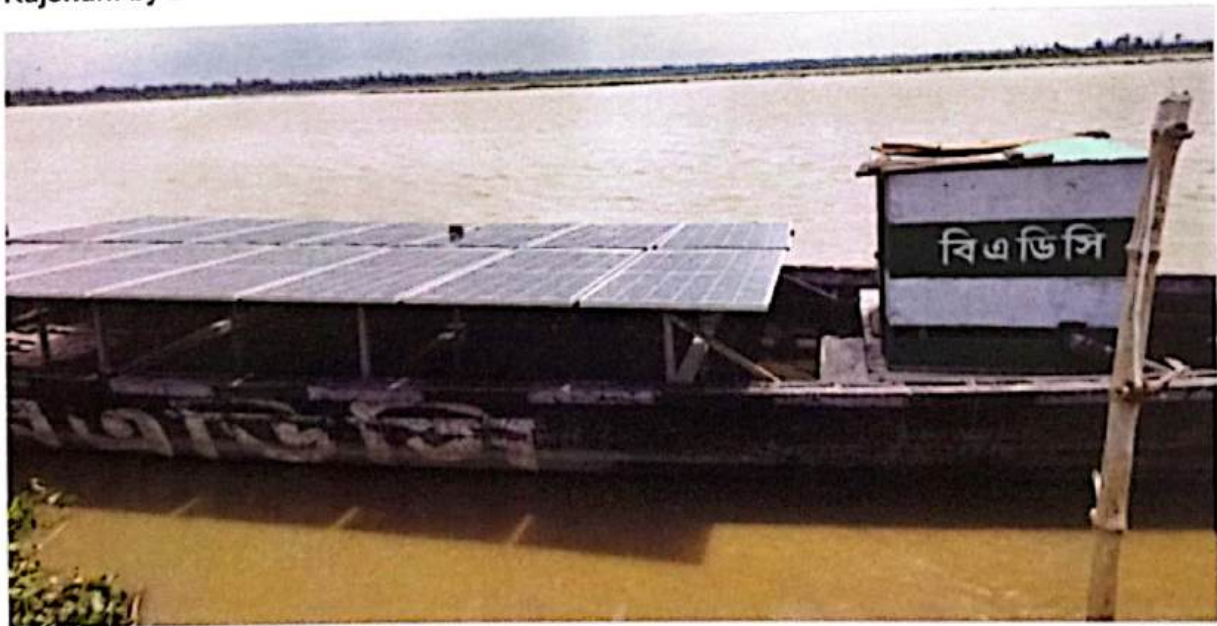
Figure 44: Boat Mounted Floating Solar LLP at Tista River, Kaunia, Rangpur by BADC
