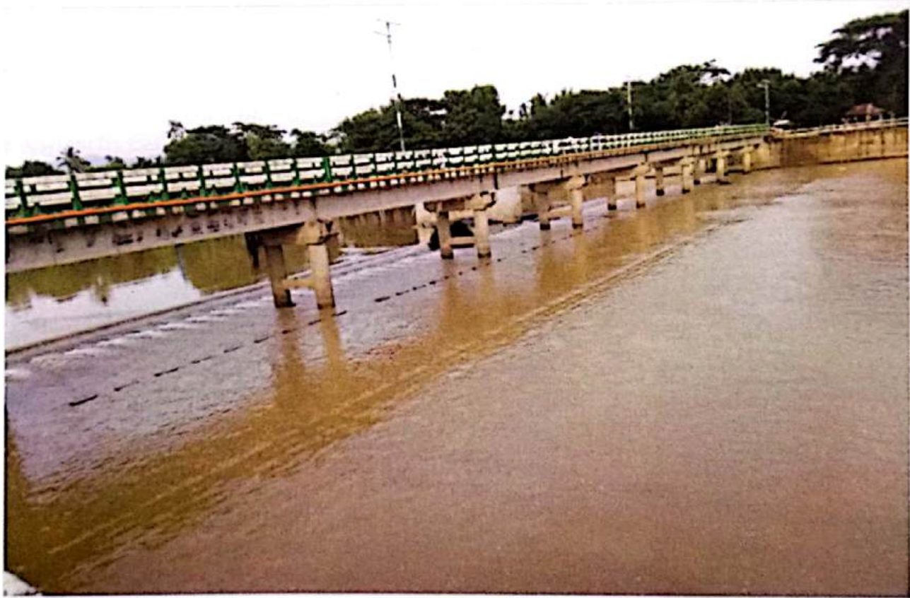
Figure 35: Rubber Dam at Kalmakanda Upazila, Netrokona District by BADC
