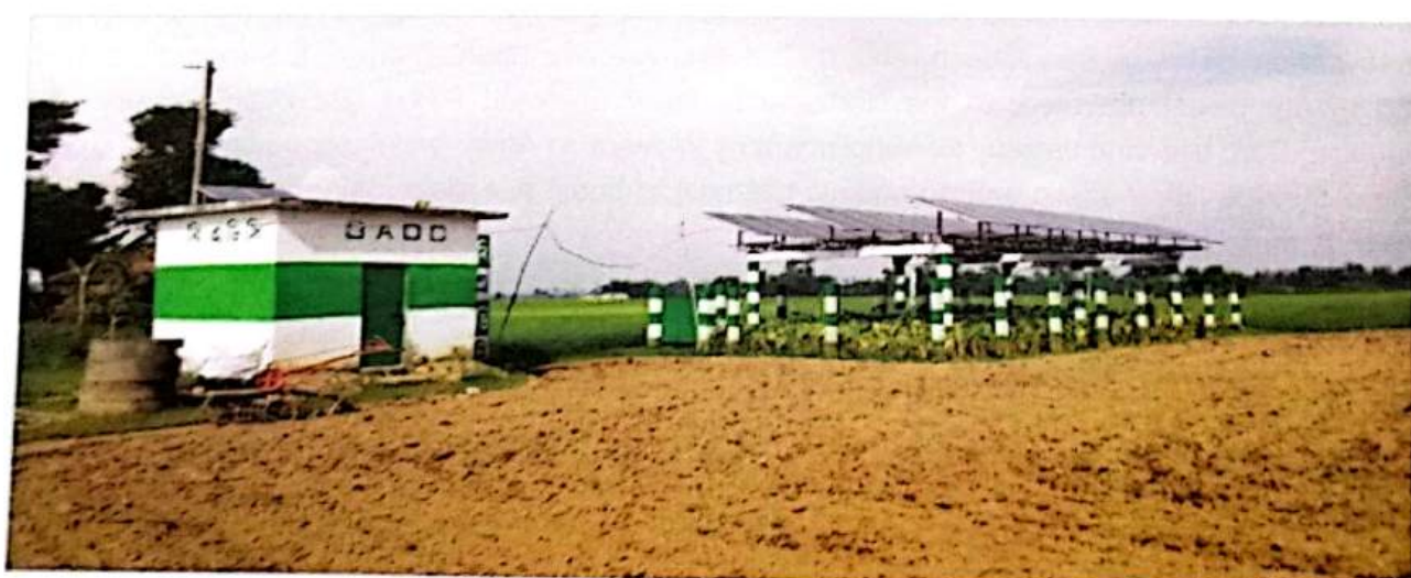
Figure 8: BADC Solar Deep Tubewell at Sadar Upazila, Sylhet
