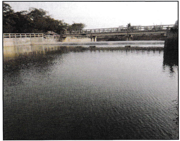
Figure 22: Chilai River Rubber Dam Doyarabazar Sunamganj
