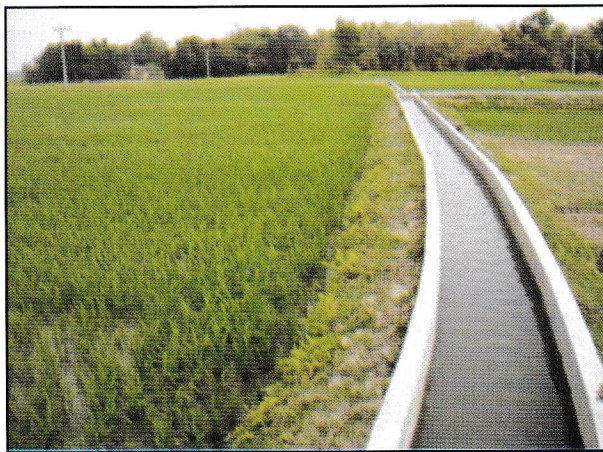
Figure 25: RCC Channel of Habiganj
