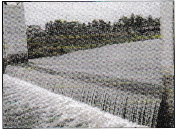
Figure 24: Submerged Weir, B. Baria
