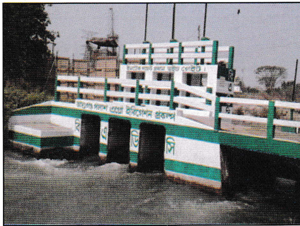
Figure 23: Intake Point Sluice Gate, B. Baria
