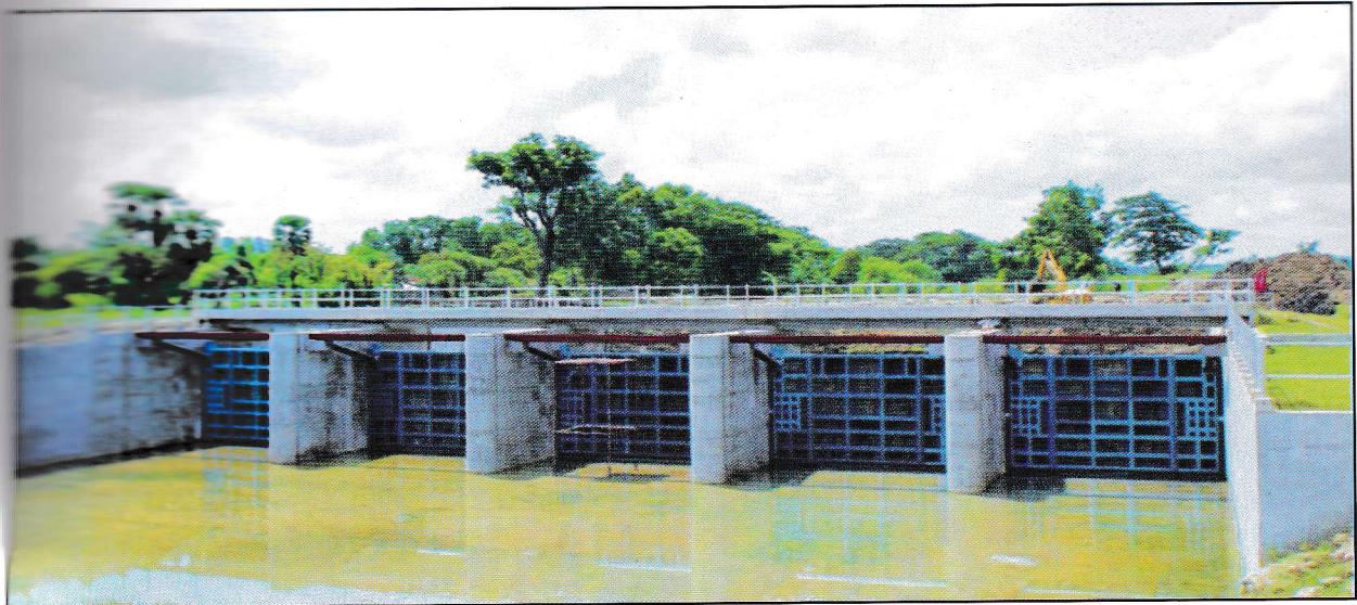
Figure 18: Hydraulic Elevated Dam in Anowara, Chottogram.
