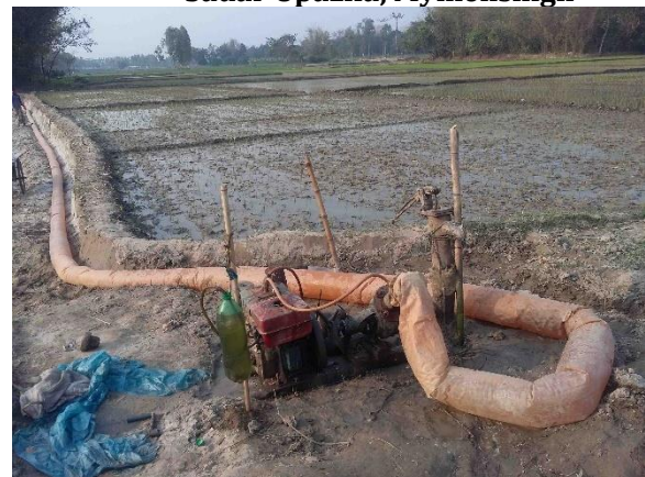
Figure 5.48: Shallow Tubewell with Fita pipe at Sadar Upazila, C. Nawabganj
