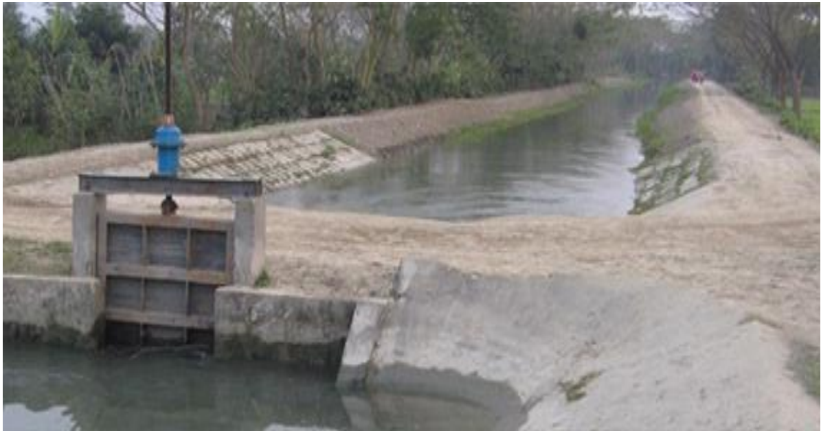
Figure 5.28: Gravity Flow Irrigation at Tista Barrage at Nilphamari by BWDB
