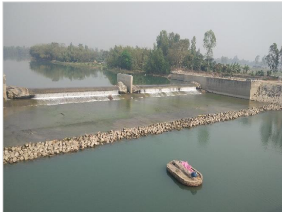
Figure 5.24: Mohanpur Rubber Dam at Sadar upazila, Dinajpur by LGED.
