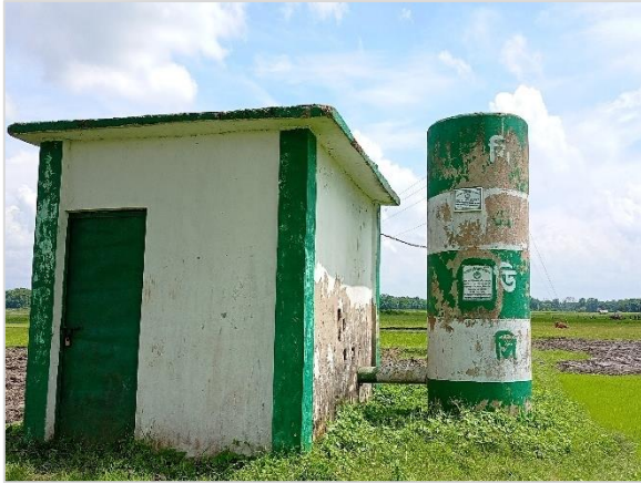
Figure 5.37: BADC Deep Tubewell at Lakhai Upazila, Habiganj
