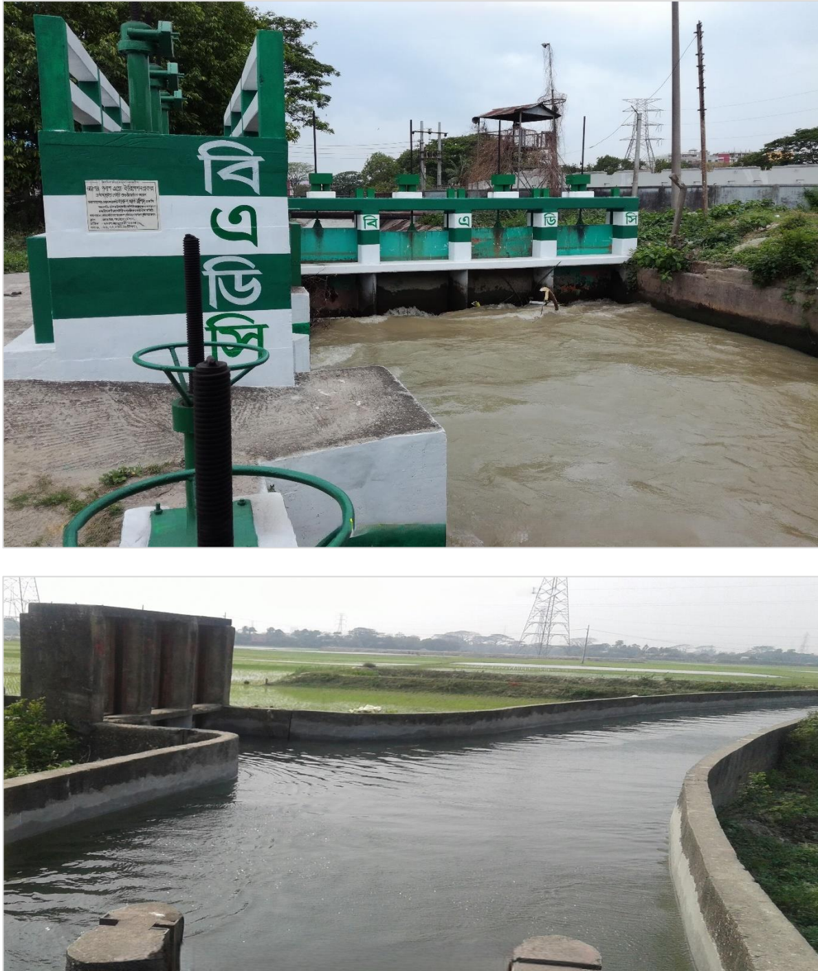
Figure 5.27: Gravity flow irrigation at Ashuganj-Polash agro-irrigation project by BADC
