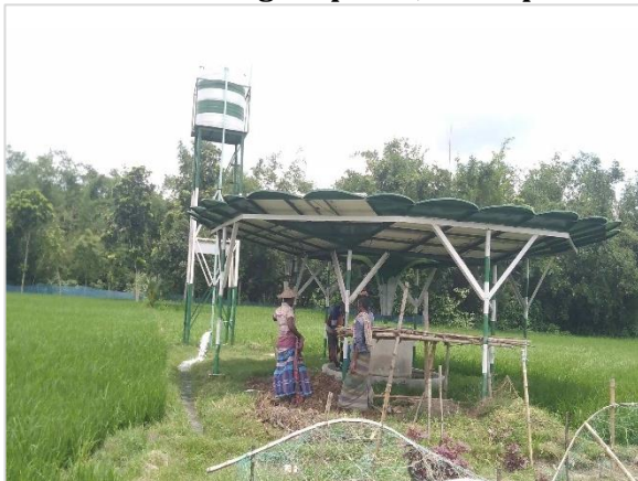
Figure 5.53: BADC Solar operated Dug well at Alamdanga, Chuadanga.
