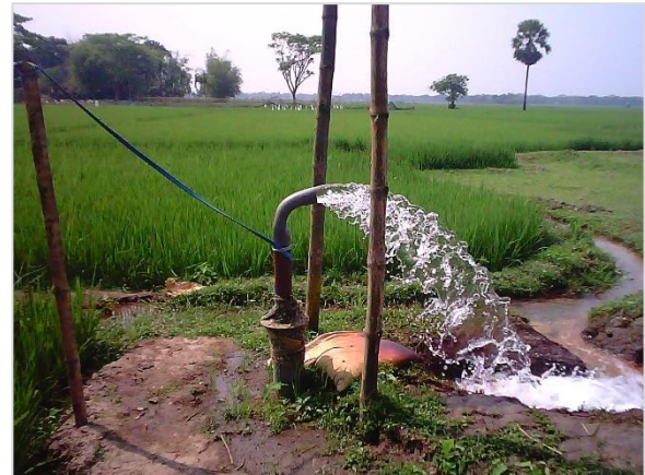
Figure 5.46: Electrified Shallow Tubewell at Sadar Upazila, Mymenshig
