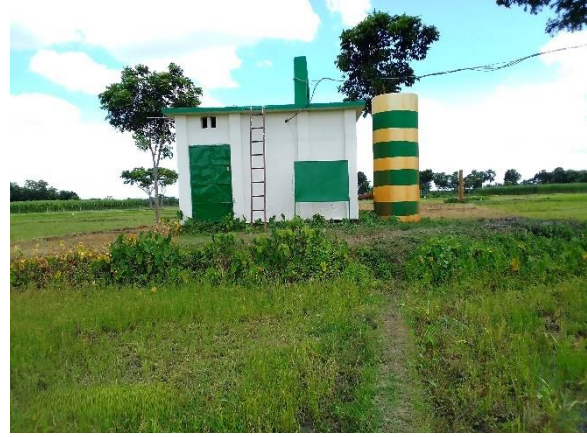
Figure 5.35: BADC Deep Tubewell at Damurhuda Upazila, Chuadanga
