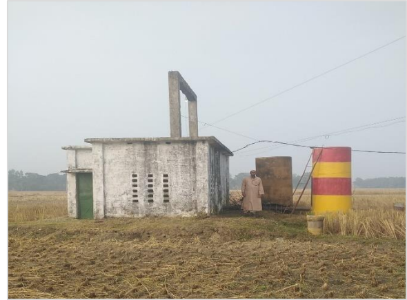
Figure 5.38: BMDA DTW in Baliadangi Upazila, Thakurgaon
