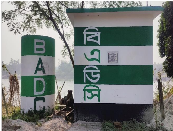
Figure 5.9: LLP with Buried Pipe, Sadar Upazila, Manikganj by BADC
