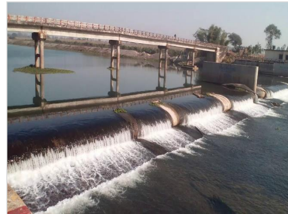
Figure 5.25: Pekua Rubber Dam at Pekua Upazila, Cox's bazar by BWDB.
