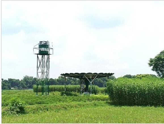
Figure 5.51: BADC Solar operated Dug well at Gangni Upazila, Meherpur
