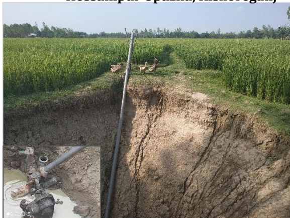
Figure 5.47: Shallow Tubewell (pit) at Patnitola Upazila, Naogaon
