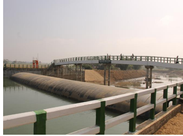
Figure 5.23: Sonai River Rubber Dam at Chatak, Sunamganj by BADC
