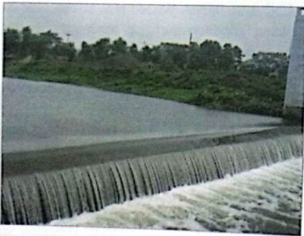
Figure 31: Submerged Weir at Ashuganj-Palash Agro Irrigation Project
