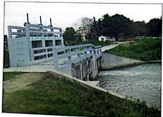
Figure 32: Intake point of Regulator at Ashuganj-Palash Agro Irrigation Project
