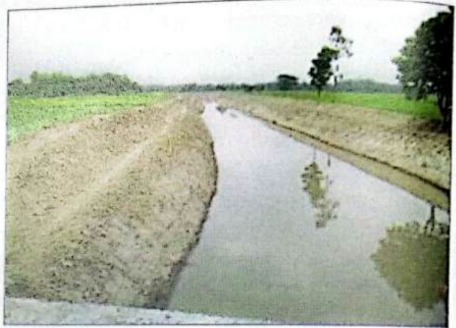
Figure 30: Re-excavated Khal at Khaliaghuri Upazila, Netrokona
