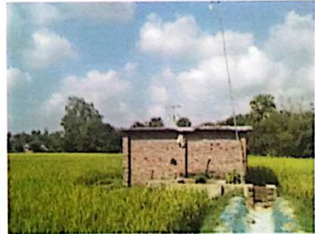
Figure 12: Private DTW at Monirampur Upazila, Jashore
