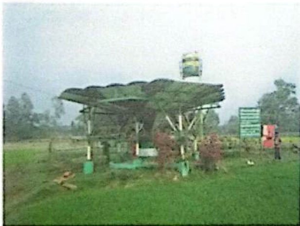
Figure 20: BADC Solar operated Dug well in Nalitabari Upazila, Sherpur District.
