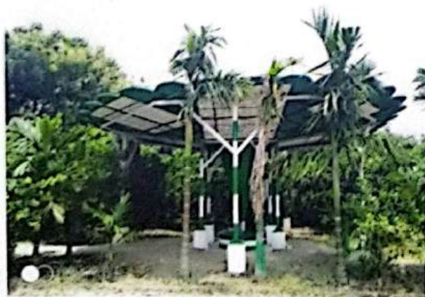
Figure 22: BADC Solar operated Dug well in Mujibnagar, Meherpur District.
