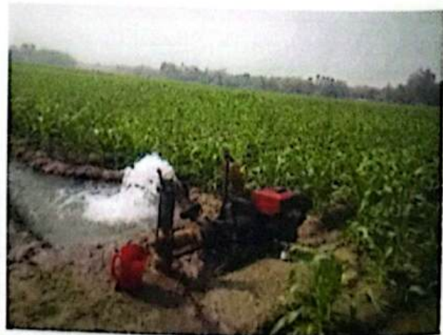
Figure 18: Shallow Tubewell at Khetlal Upazila, Joypurhat
