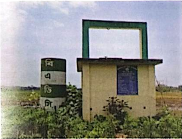
Figure 9: BADC DTW in Kalaroa Upazila, Satkhira
