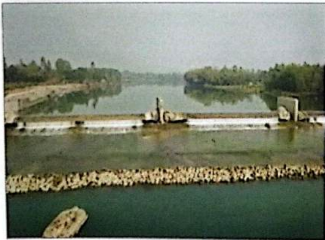
Figure 45: Rubber Dam on Atrai river at Mohonpur upazila, Dinajpur by LGED.
