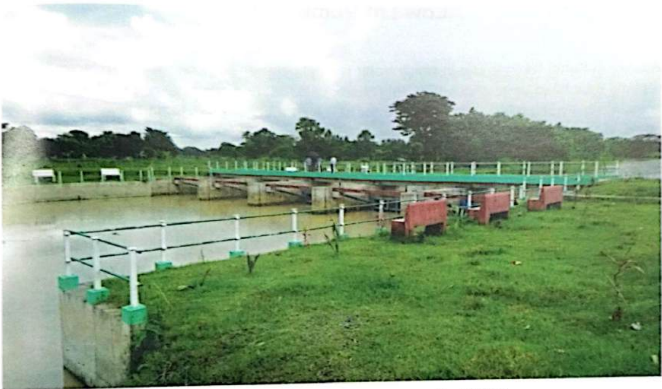
Figure 33: Hydraulic Elevated Dam at Anwara, Chattogram by BADC
