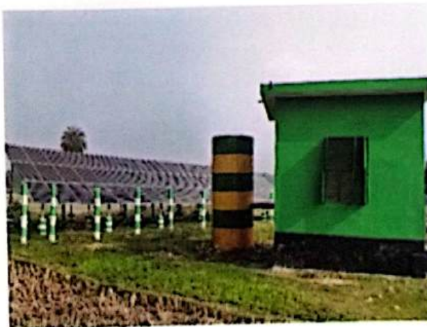
Figure 13: BADC Solar DTW at Sadar Upazila, Jashore
