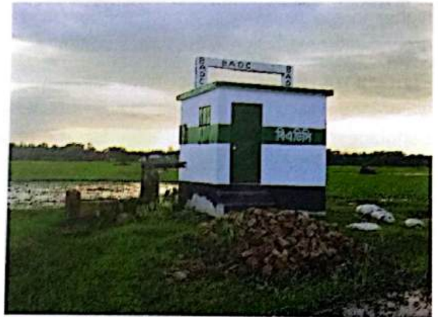
Figure 7: BADC Deep Tubewell at Kosba Upazila, Brahmanbaria
