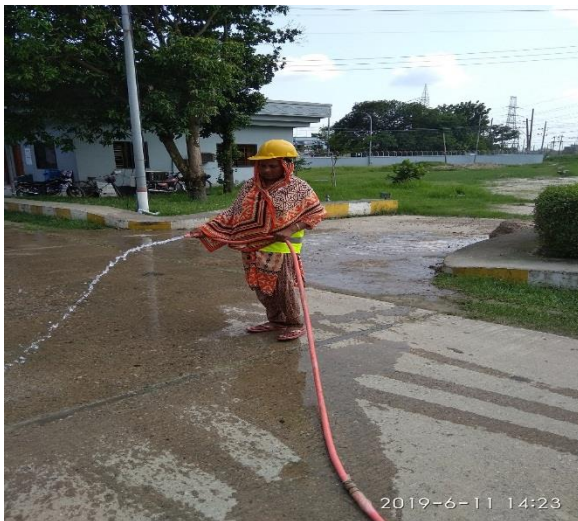
Figure 4.15: Water is sprinkled for dust control
