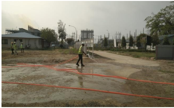
Water Spraying for dust control
