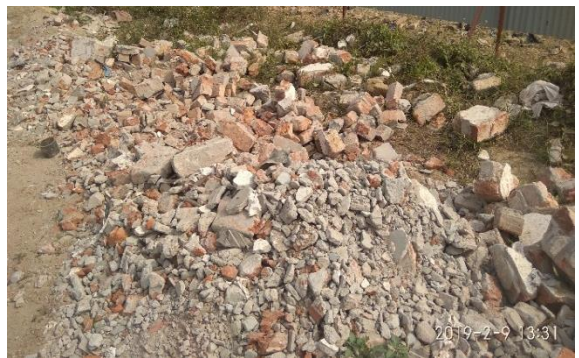
Boundary Demolition at the end stage
