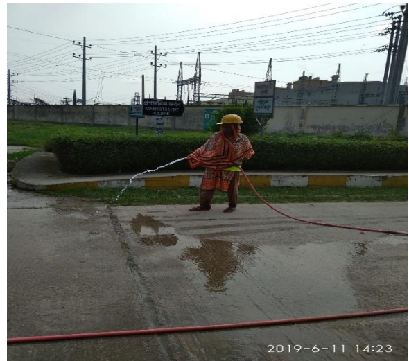
Figure 4.15: Water is sprinkled for dust control
