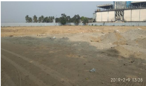
Site condition of February
