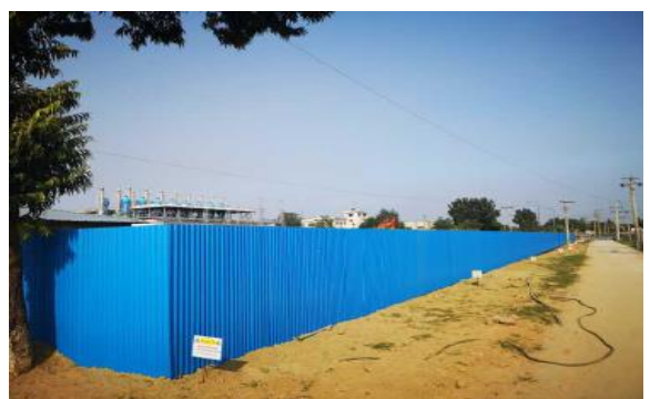
Fencing at site
