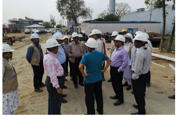
Site visit by high officials of Ministry of Power, Energy & Mineral Resources
