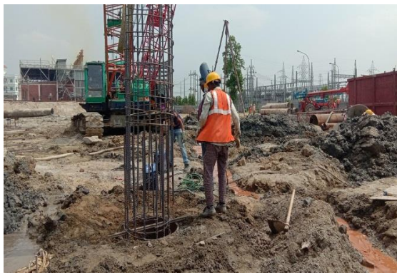
Piling activity- rebar cage
