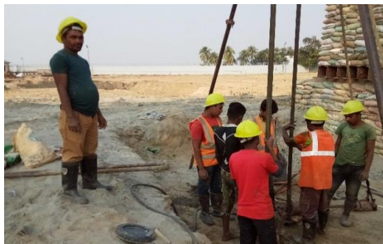
Workers with proper PPE
