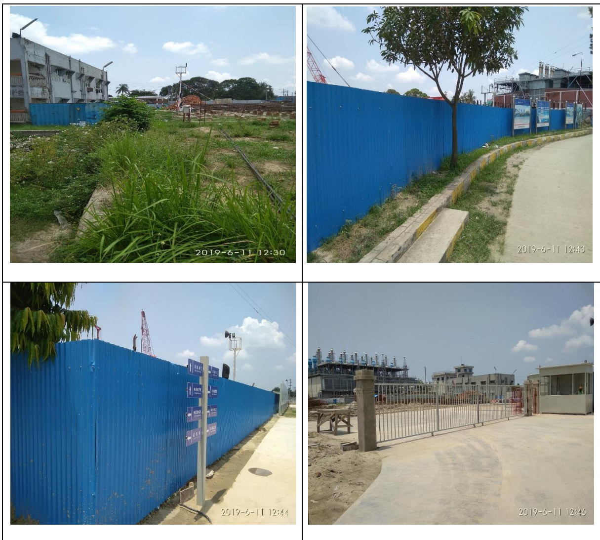
Figure 4.6: Present Fencing Conditions of the Project Site
