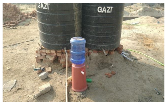
On site drinking water facility
