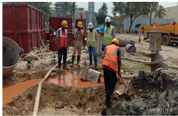
Piling activity- Flashing
