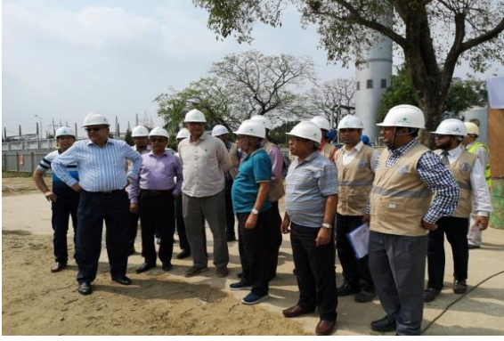
Site visit by high officials of Ministry of Power, Energy & Mineral Resources
