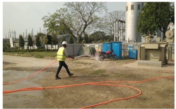
Water Spraying for dust control
