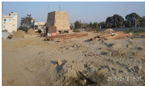
Pile test period in February
