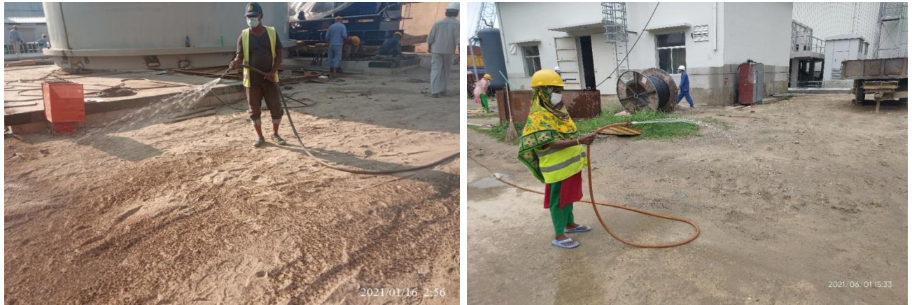
Figure 10: Water is spraying for dust control
