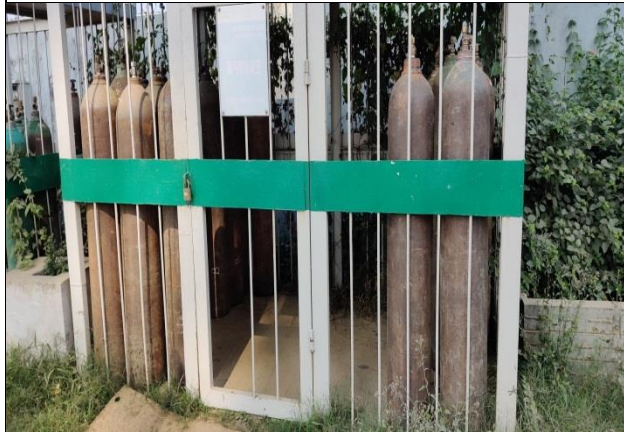
Safe Storage of Pressurized Gas Cylinders
