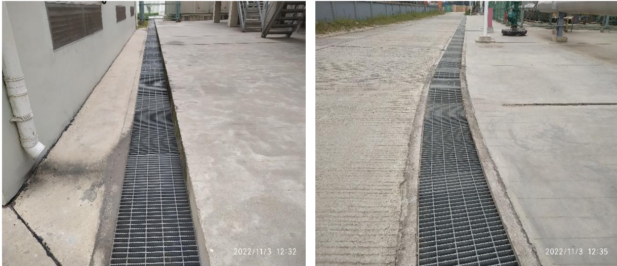
Figure 20: Photograph of Site Drainage
