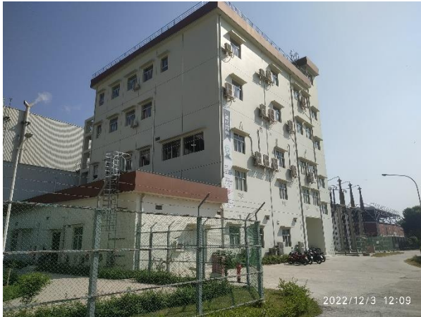
Central Control Building (CCB)
