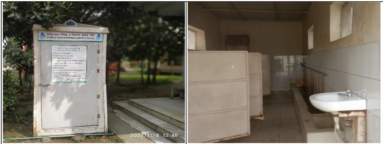
Figure 19: Pure Drinking Water & Sanitation facility to workers
