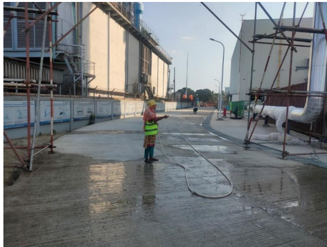
Figure 22: Water spraying for dust control
