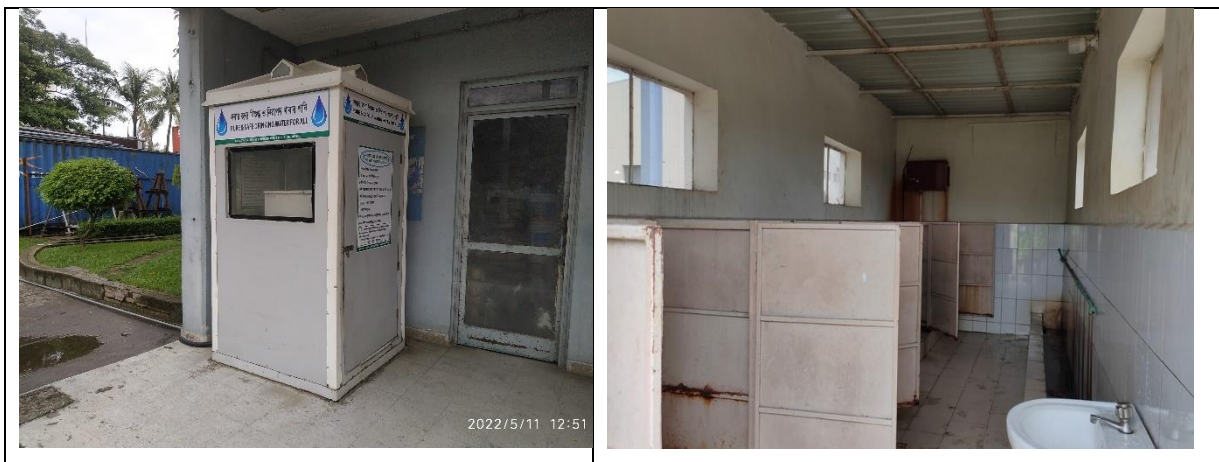
Figure 20: Pure Drinking Water & Sanitation facility to workers
