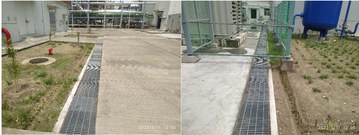
Figure 21: Photograph of Site Drainage
