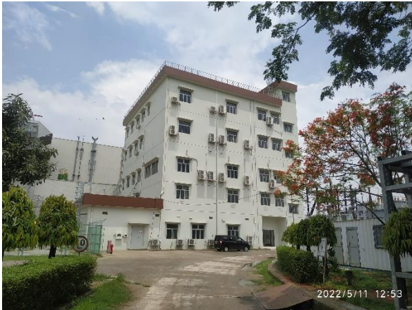
Fig. 1.2.1: Construction of Central Control Building (CCB)
