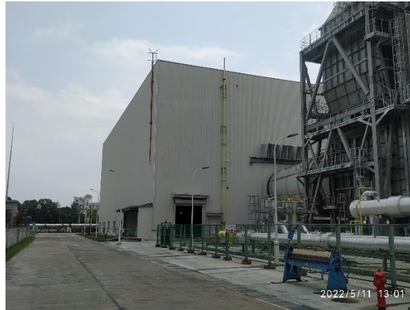
Fig.1.2.2: Construction of main building
