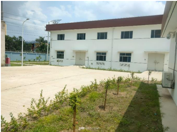
Fig. 1.2.4: Construction of chemical plant & Plantation at site
