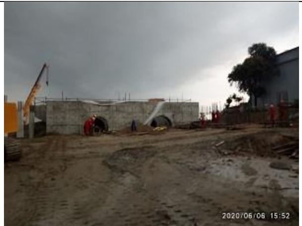
Fig: Construction of water intake plant
