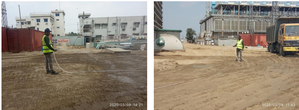
Figure -15: Water is spraying for dust control
