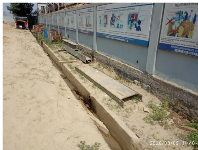
Figure-14: Existing outer drainage and rainy water reservoir
