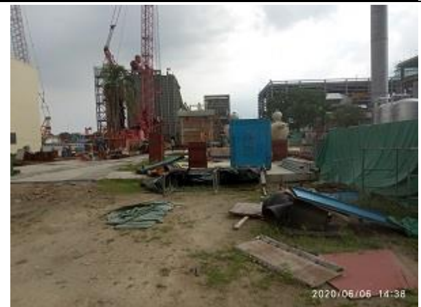
Fig: Construction of RMS Building
