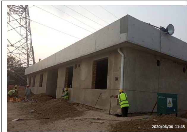
Fig: Construction of chemical plant
