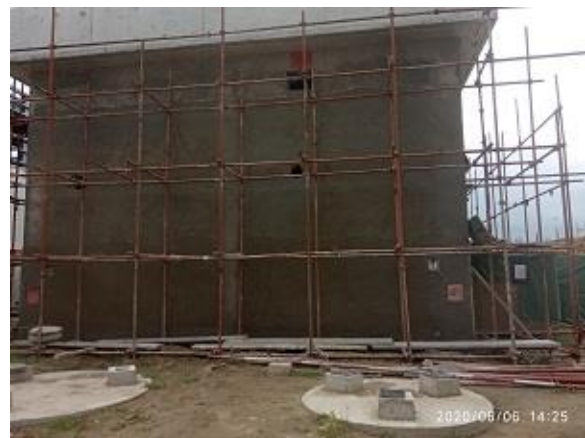
Fig: Construction of oily waste water treatment station and service fire water tank
