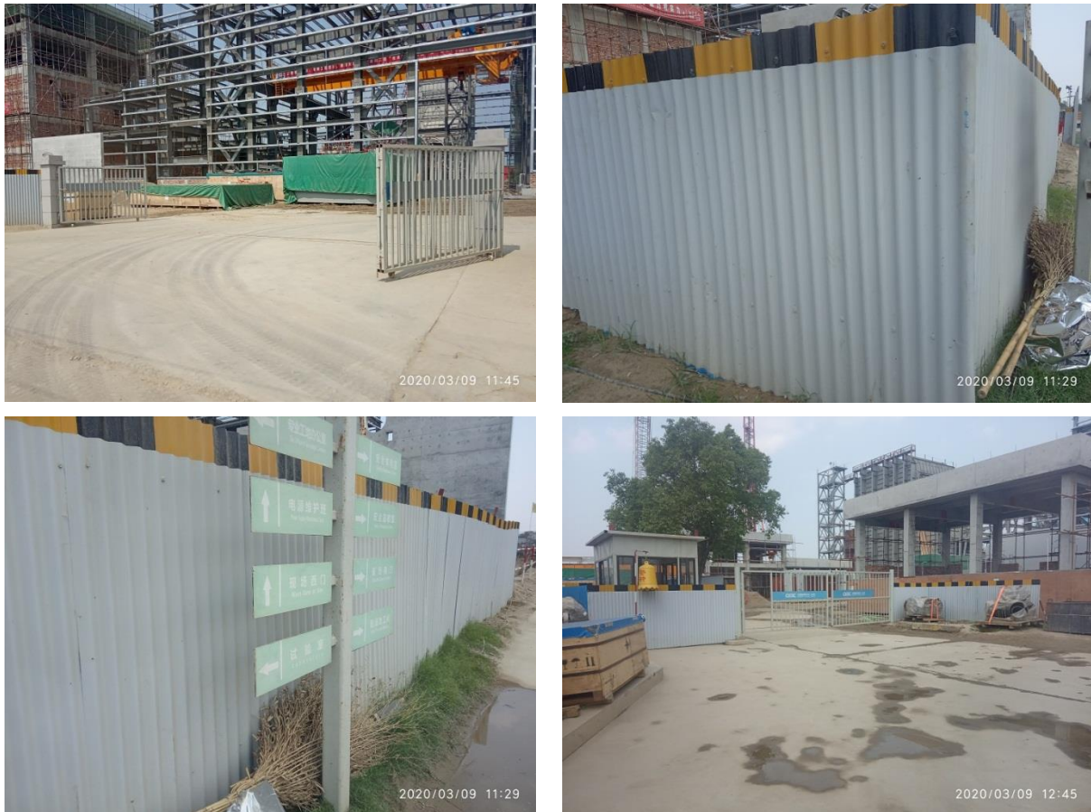
Figure-5: Present fencing conditions of the Project Site
