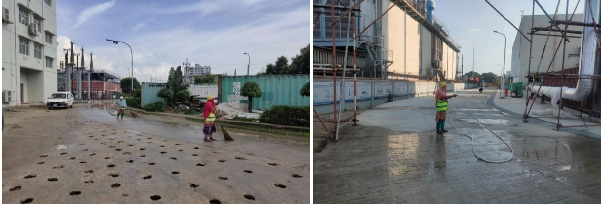
Figure 10: Water is spraying for dust control
