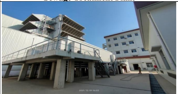
Power Control Center
