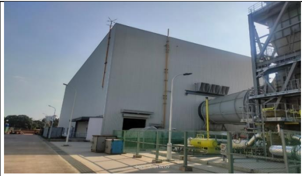
Construction of Turbine-Generator Hall
