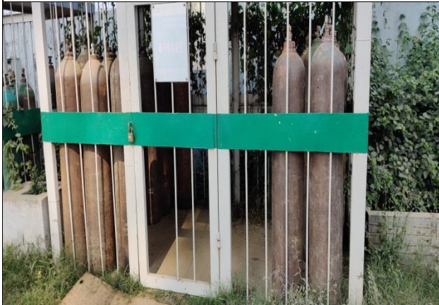
Safe Storage of Pressurized Gas Cylinders
