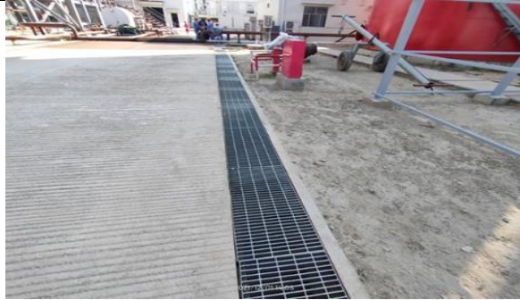
Road and Drainage System
