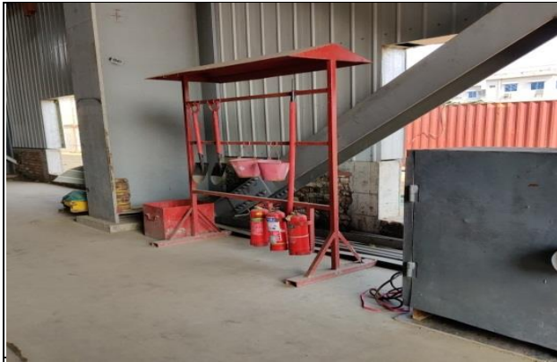
On-site Firefighting Appliances
