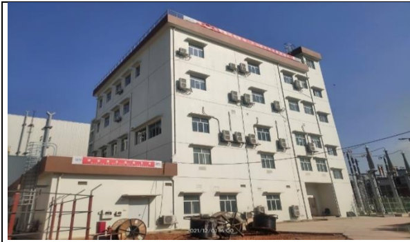
Construction of Central Control Building
