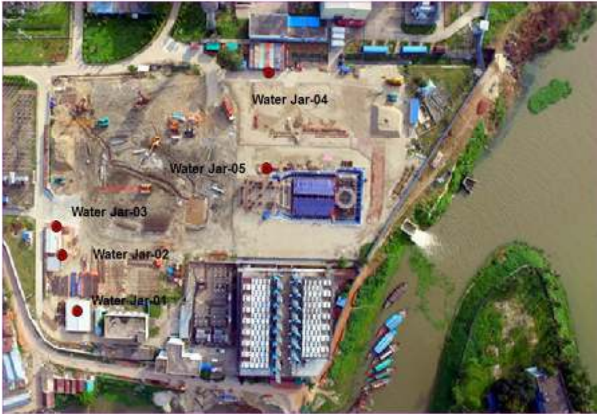
Figure 4.15: Water Jar Location at Project Site
