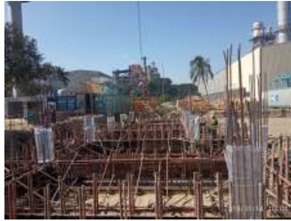
Construction of water treatment plant
