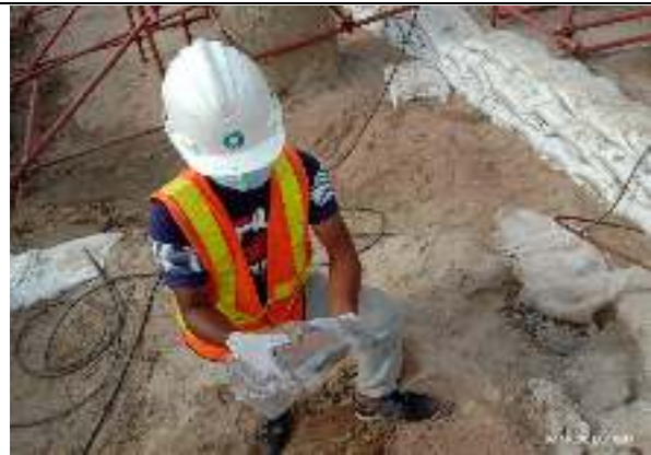
Soil Sample Collection from inside the project
