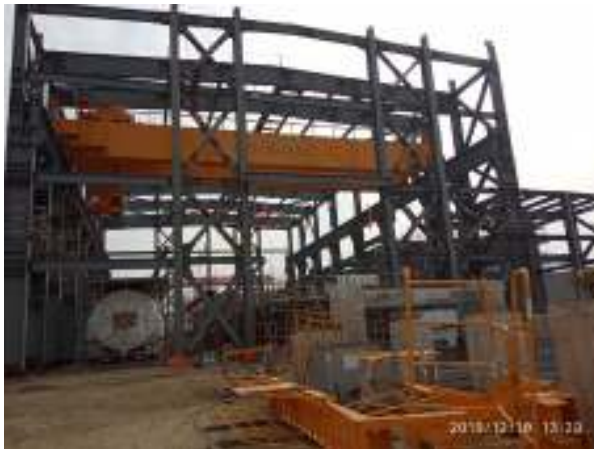
Construction of generator house
