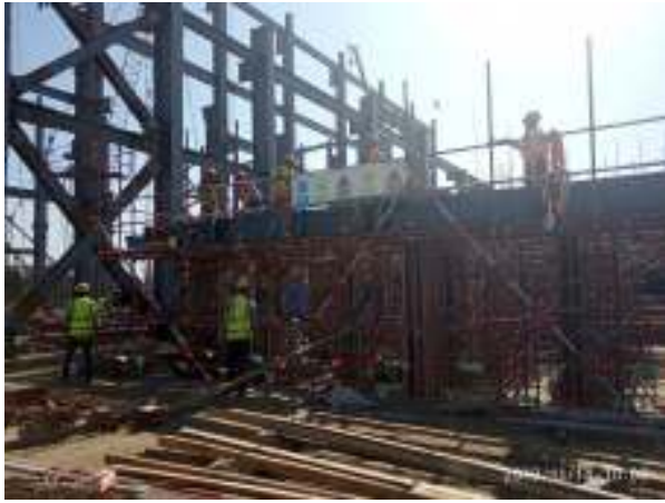
Construction of control room
