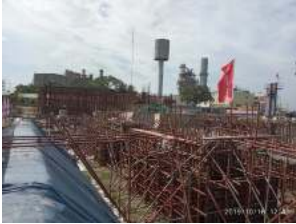
Sub structure construction work at the project site
