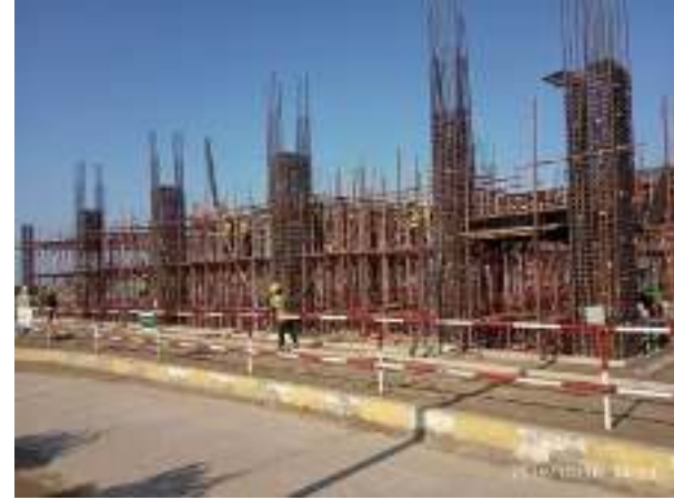
Scaffolding work for column construction at the project site
