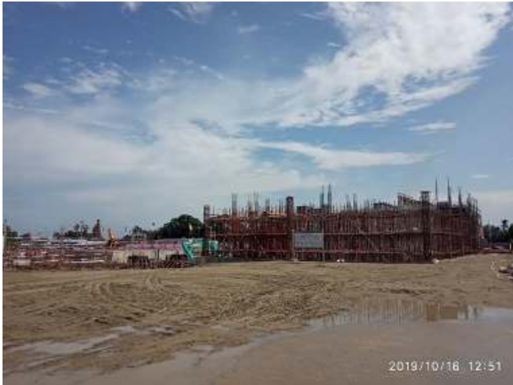
Photograph of CCB construction works at project site
