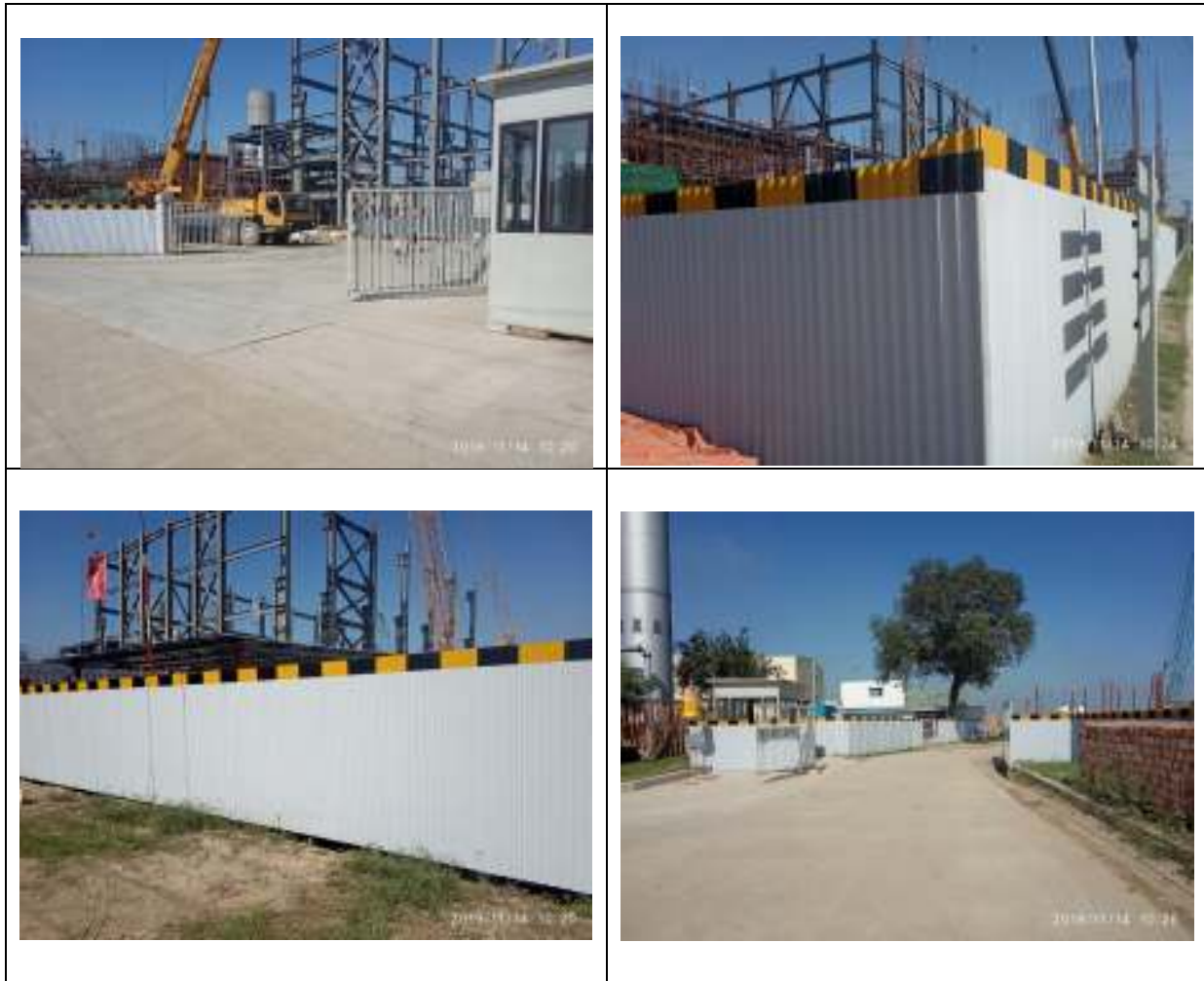
Figure 4.7: Present Fencing Conditions of the Project Site
