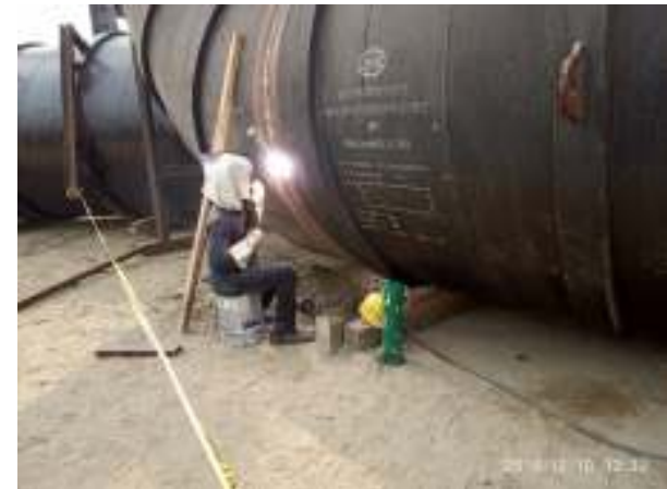
Welding work of construction site
