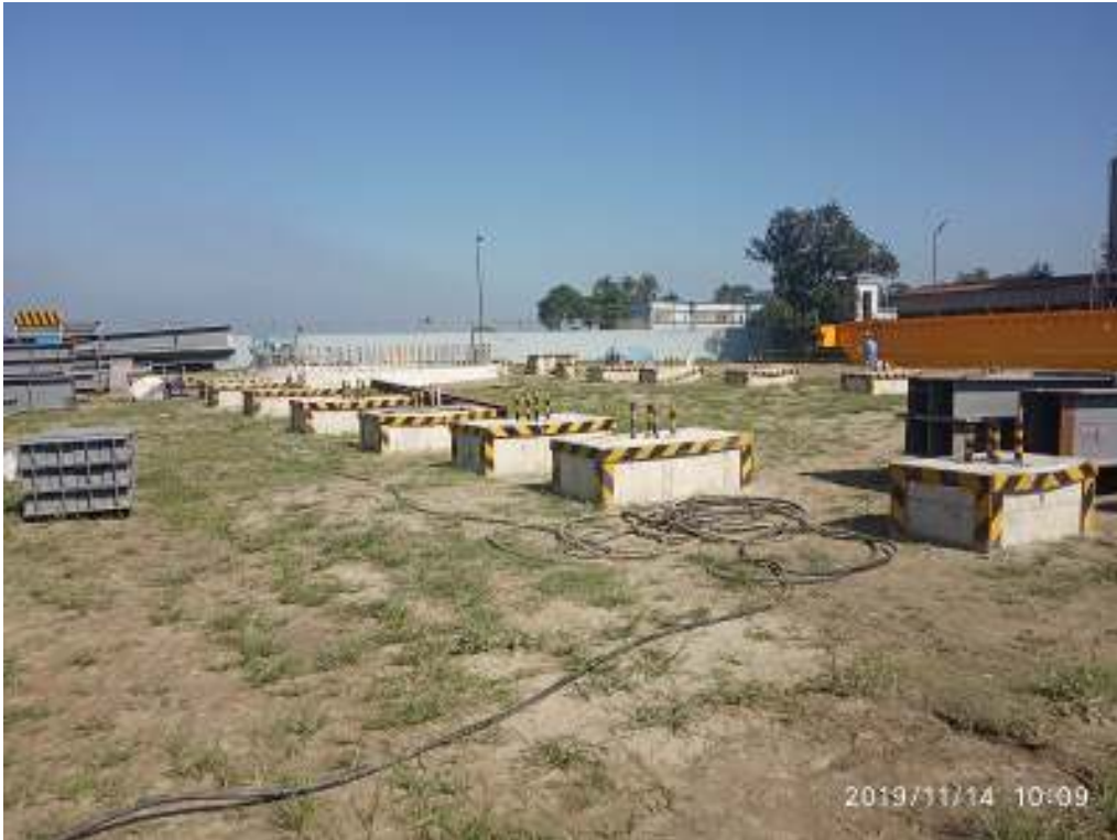
Photograph of construction works at project site
