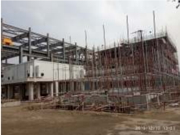
Construction of control room
