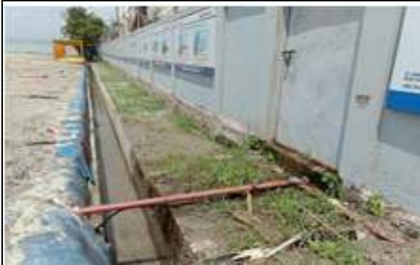
Existing outer drainage
