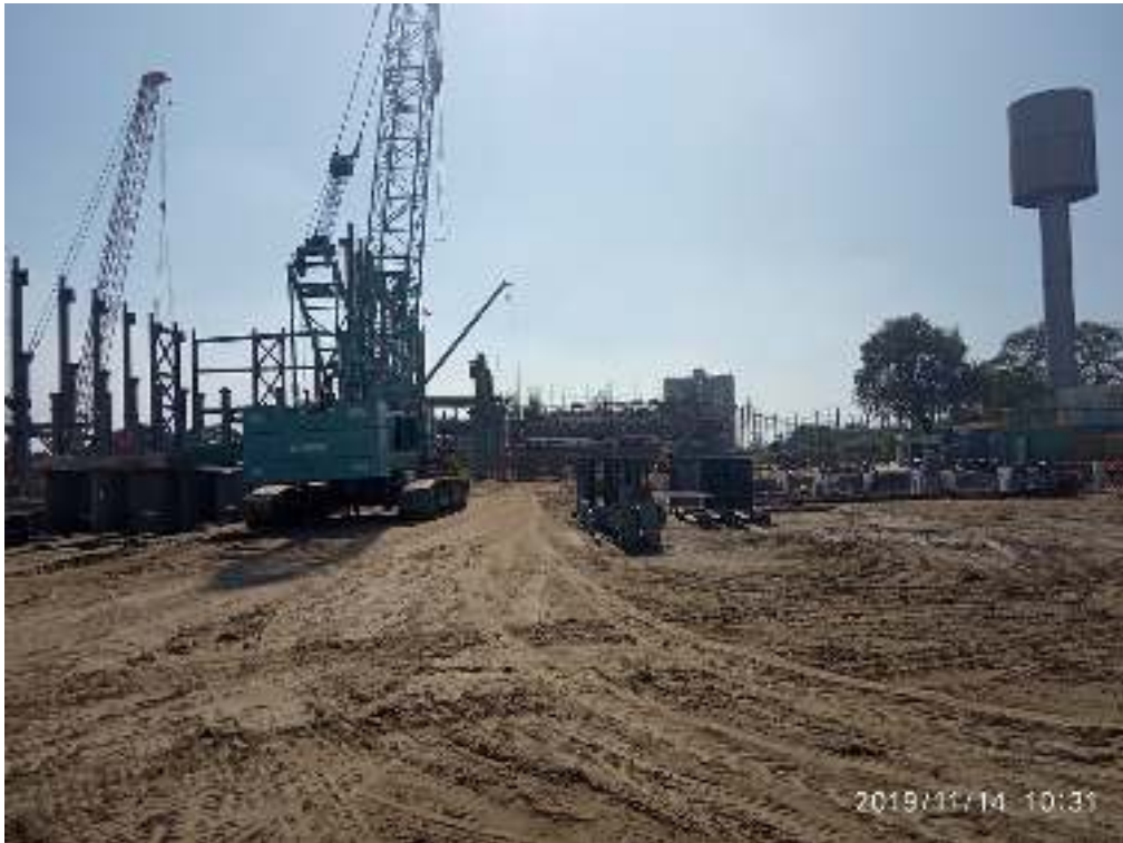
Photograph of Sub structure and Super structure construction
