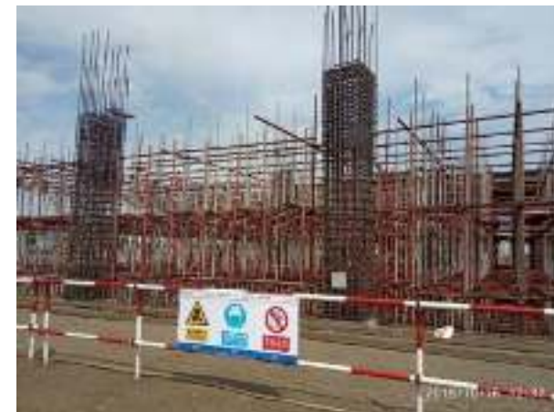
Scaffolding for construction of column at project site
