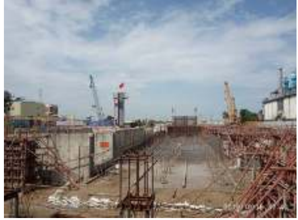
Shuttering Form work at the project site
