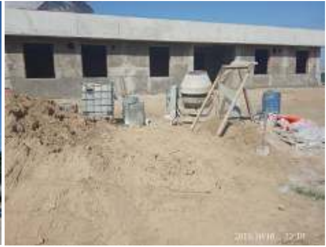
Construction of Water Treatment Plant
