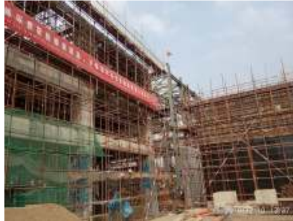
Construction of main building
