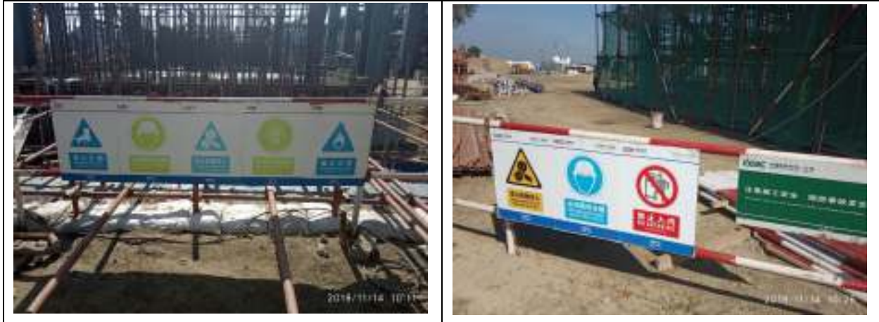
Figure 4.8: Sign Boards and Pictorial Safety at the Project Site
