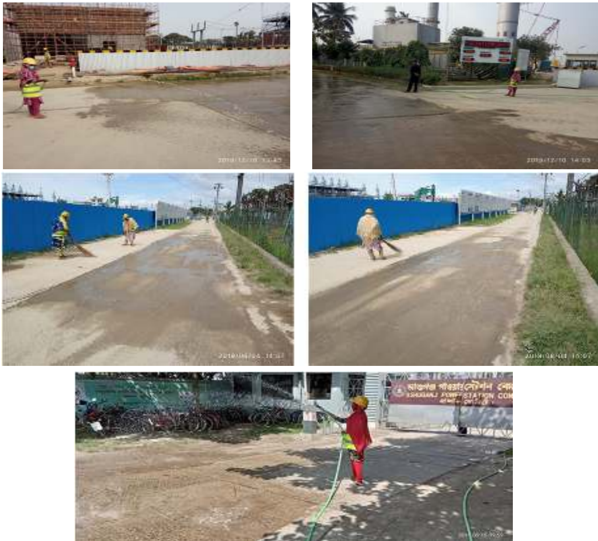
Figure 4.17: Water Spraying for Dust Control
