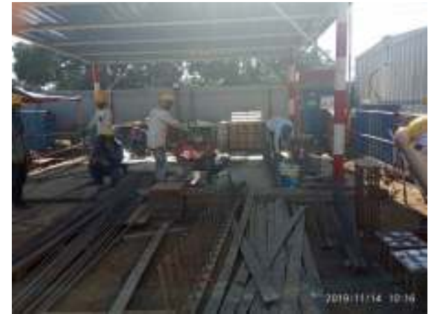
Welding work of construction site
