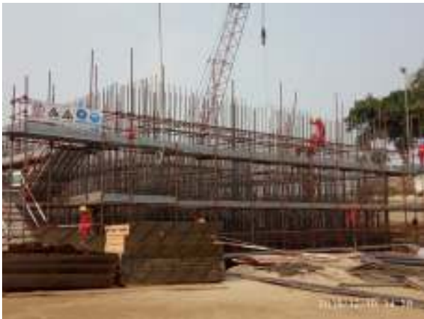
Scaffolding works of construction site
