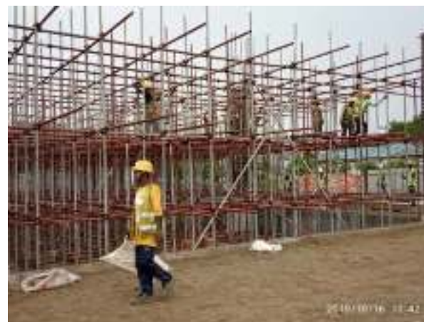
Scaffolding for construction of column at project site
