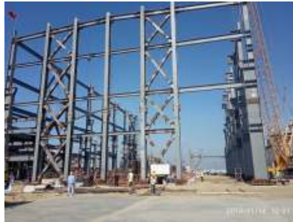
Construction of generator hall
