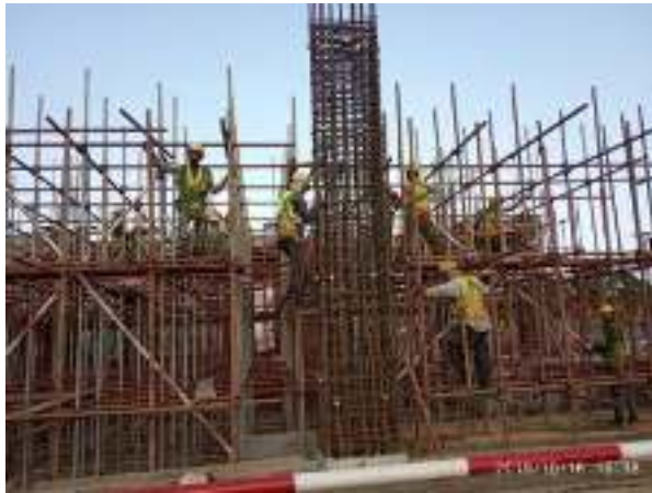
Super structure work of construction
