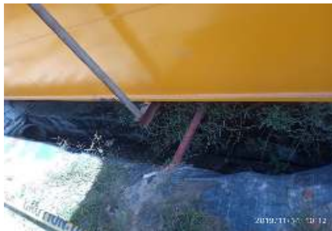
Figure 4.16: Existing Outer Drainage and Rain Water Reservoir
