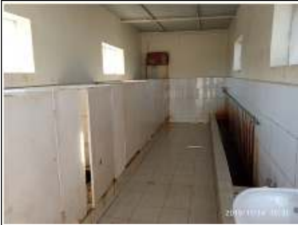
Wash Room/Sanitation Facilities
