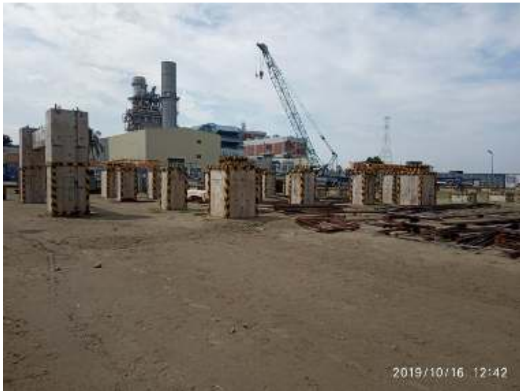
Sub structure construction has been completed in HRSG portion
