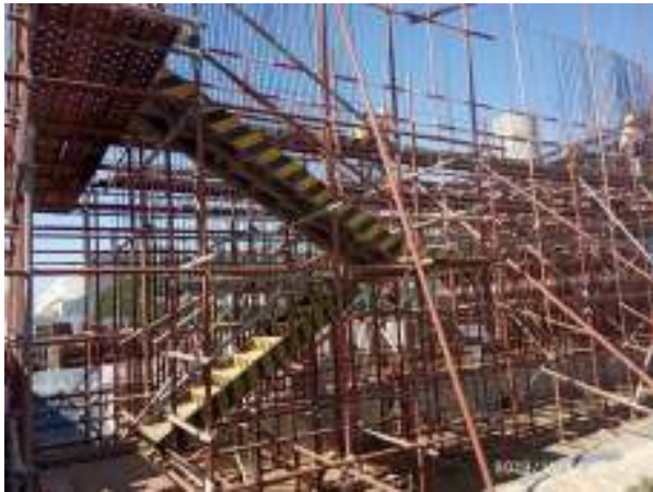
Scaffolding works of construction site
