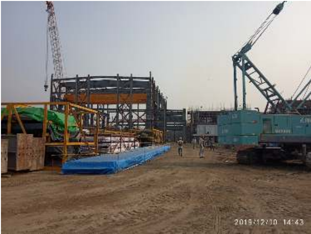
Photograph of superstructure construction of Generator Hall
