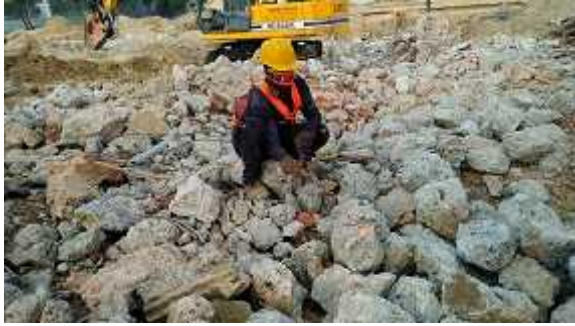
Demolition performed with proper PPE
