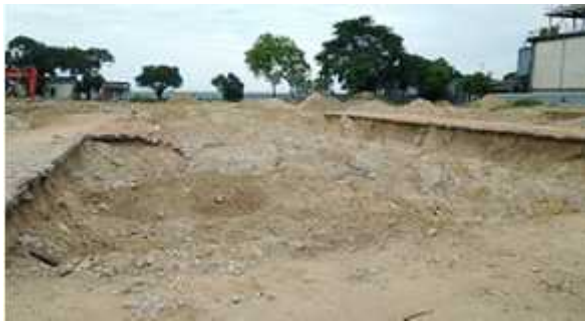
Demolition at the end stage
