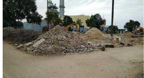
Demolition waste stored in a place
