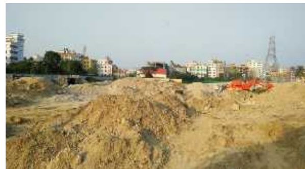
Construction Debris Storage Location
