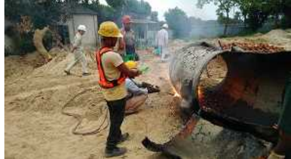
Water spraying during cutting/hot works
