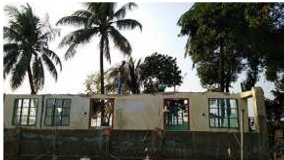
Demolition works at site
