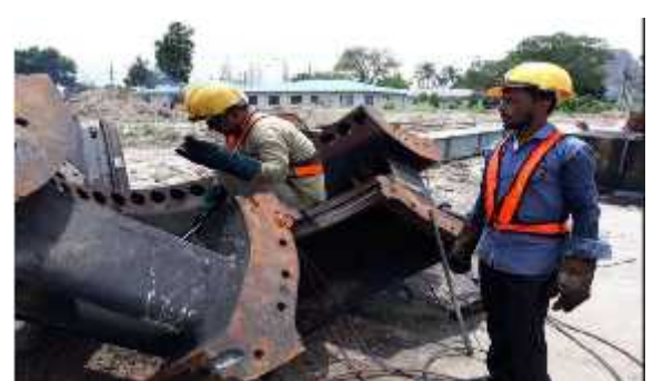
Demolition activities with proper PPE
