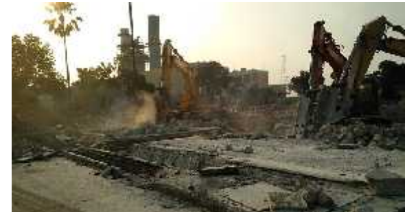
Site Demolition works
