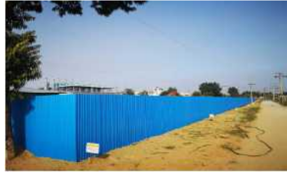
Safety Fencing at site
