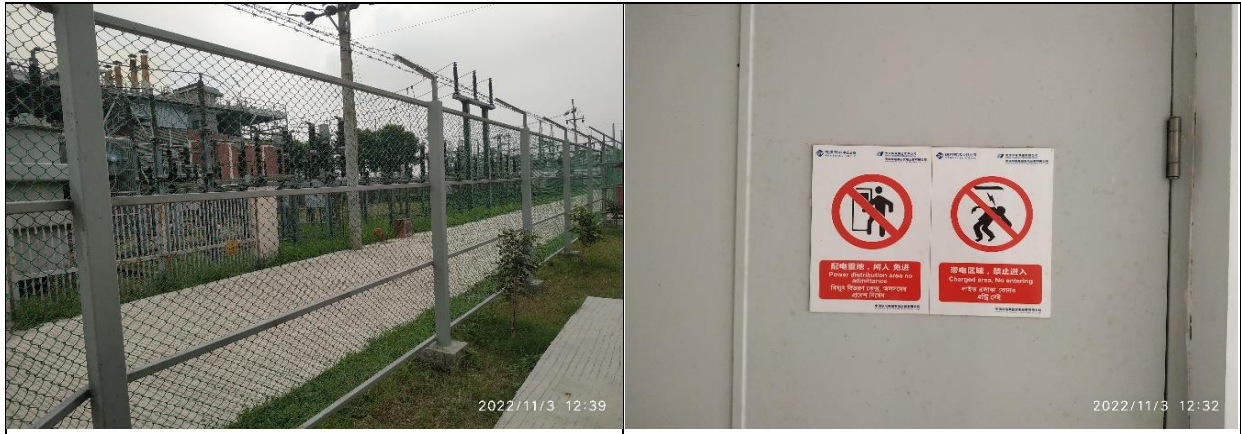
Figure 4: Site Security & Safety Instruction Board
