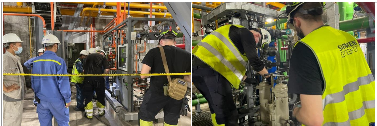
Figure 5: Use of Proper PPEs
