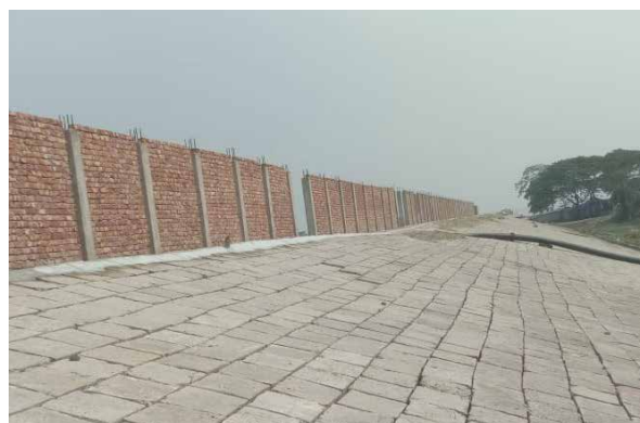
Earth Protection Work by CC Block
