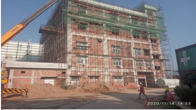
Construction of Central Control Building
