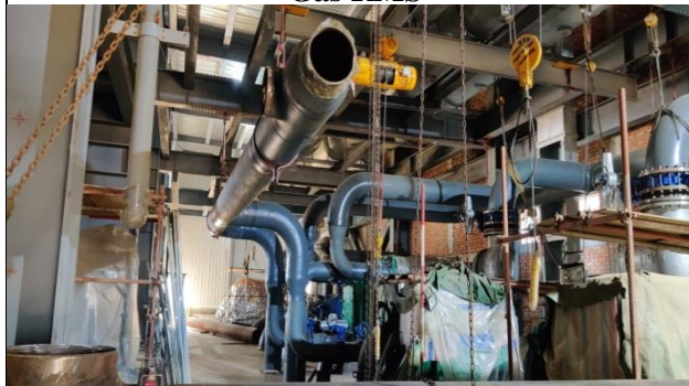
Installation of Different Auxiliaries
