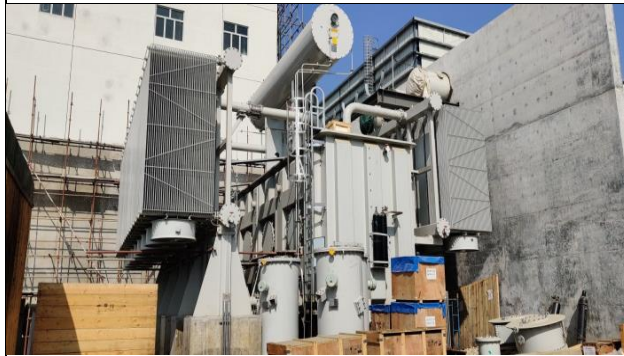
Transformer Installation
