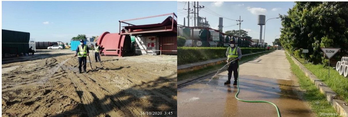
Figure 10: Water spraying for dust control
