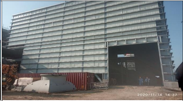
Construction of Turbine-Generator Hall
