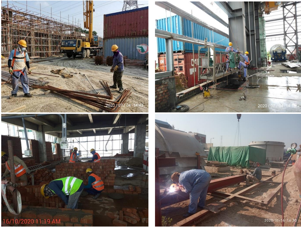
Figure 5: Use of Proper PPEs
