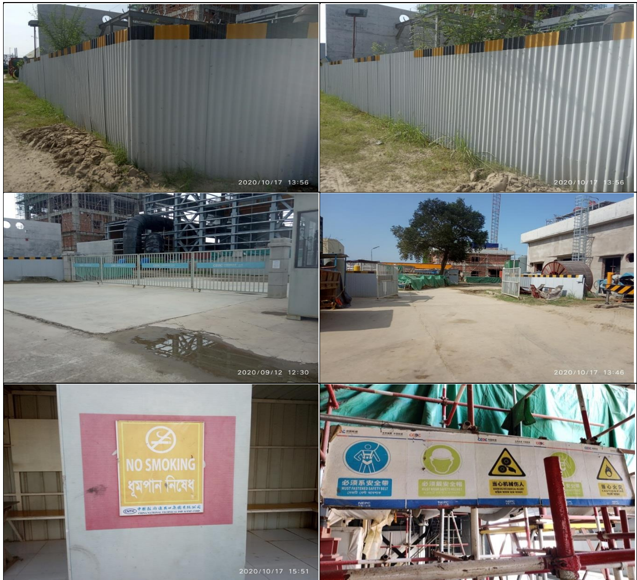
Figure 10: Site Security & Safety Instruction Board
