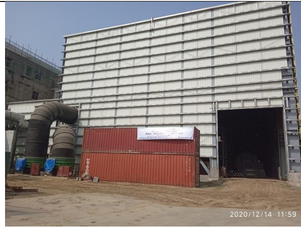
Construction of Turbine Hall
