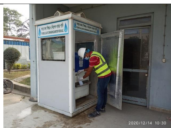
South-west side of Project area near admin building purifier (D2)
