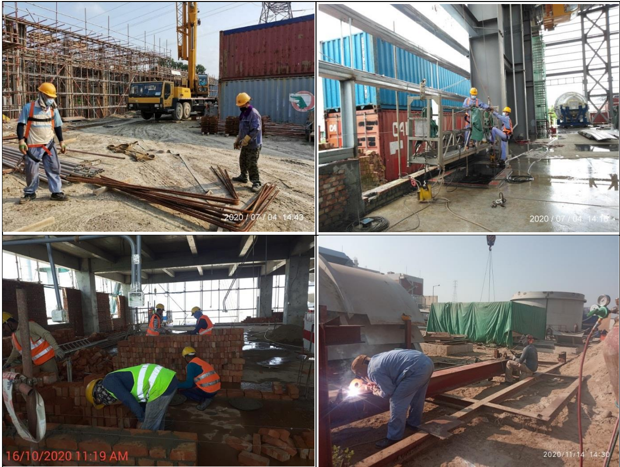
Figure 11: Use of Proper PPEs
