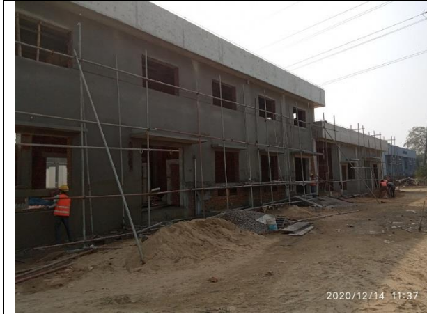
Construction of chemical plant
