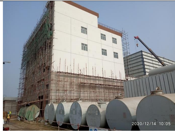
Construction of Central Control Building (CCB)
