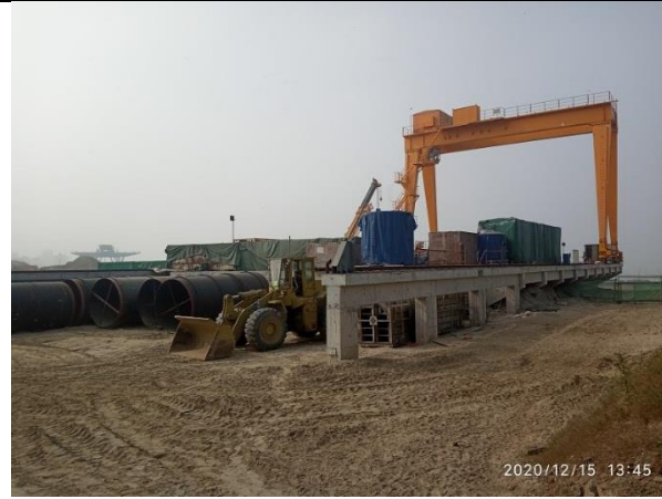
Construction of water intake plant
