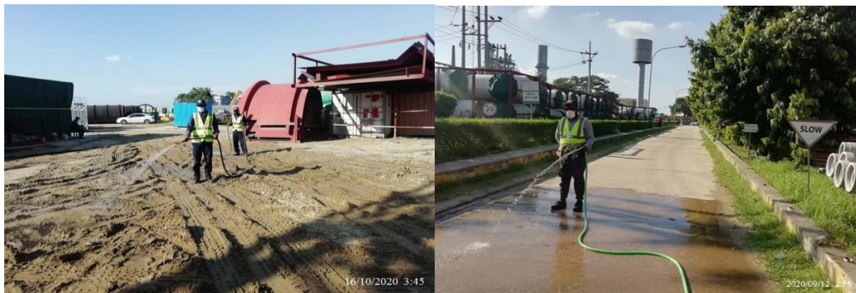
Figure 18: Water spraying for dust control
