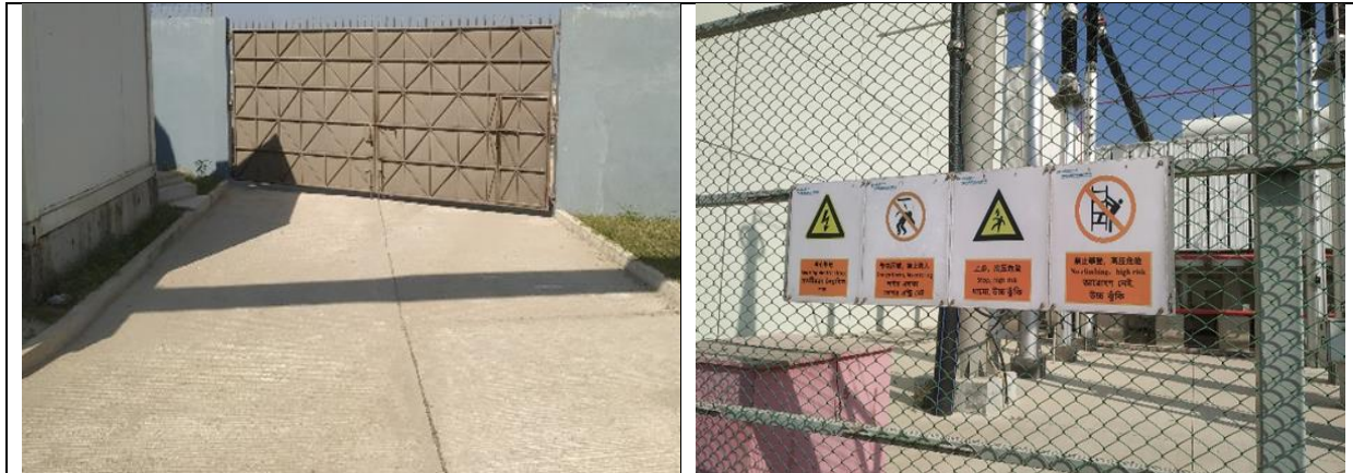
Figure 6: Present Boundary Wall Condition & Warning Signage at the Plant Site
