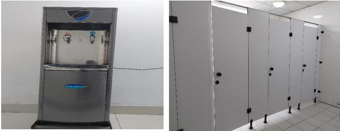
Figure 10: Pure Drinking Water & Sanitation facility to workers
