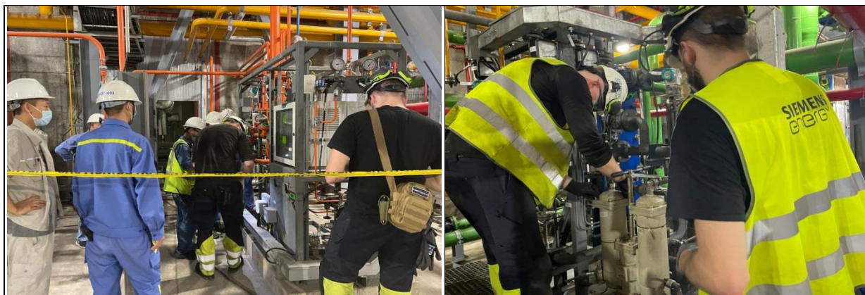
Figure 7: Use of Proper PPEs during Works
