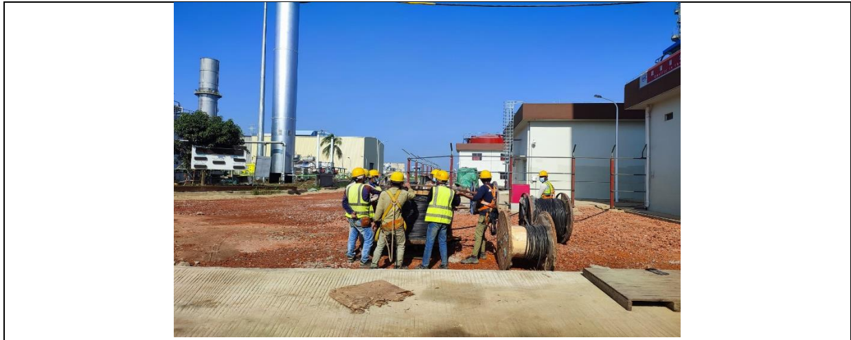
Figure 12: Use of Proper PPEs
