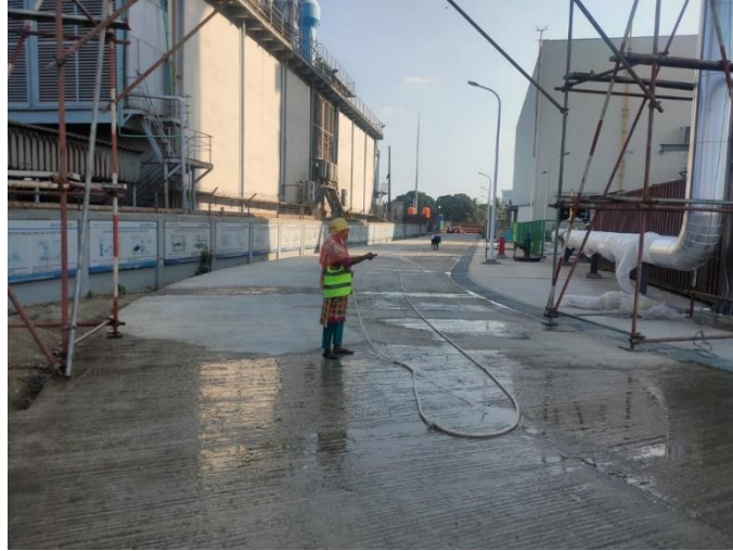
Figure 21: Water spraying for dust control
