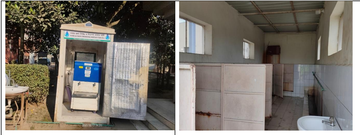
Figure 19: Pure Drinking Water & Sanitation facility to workers
