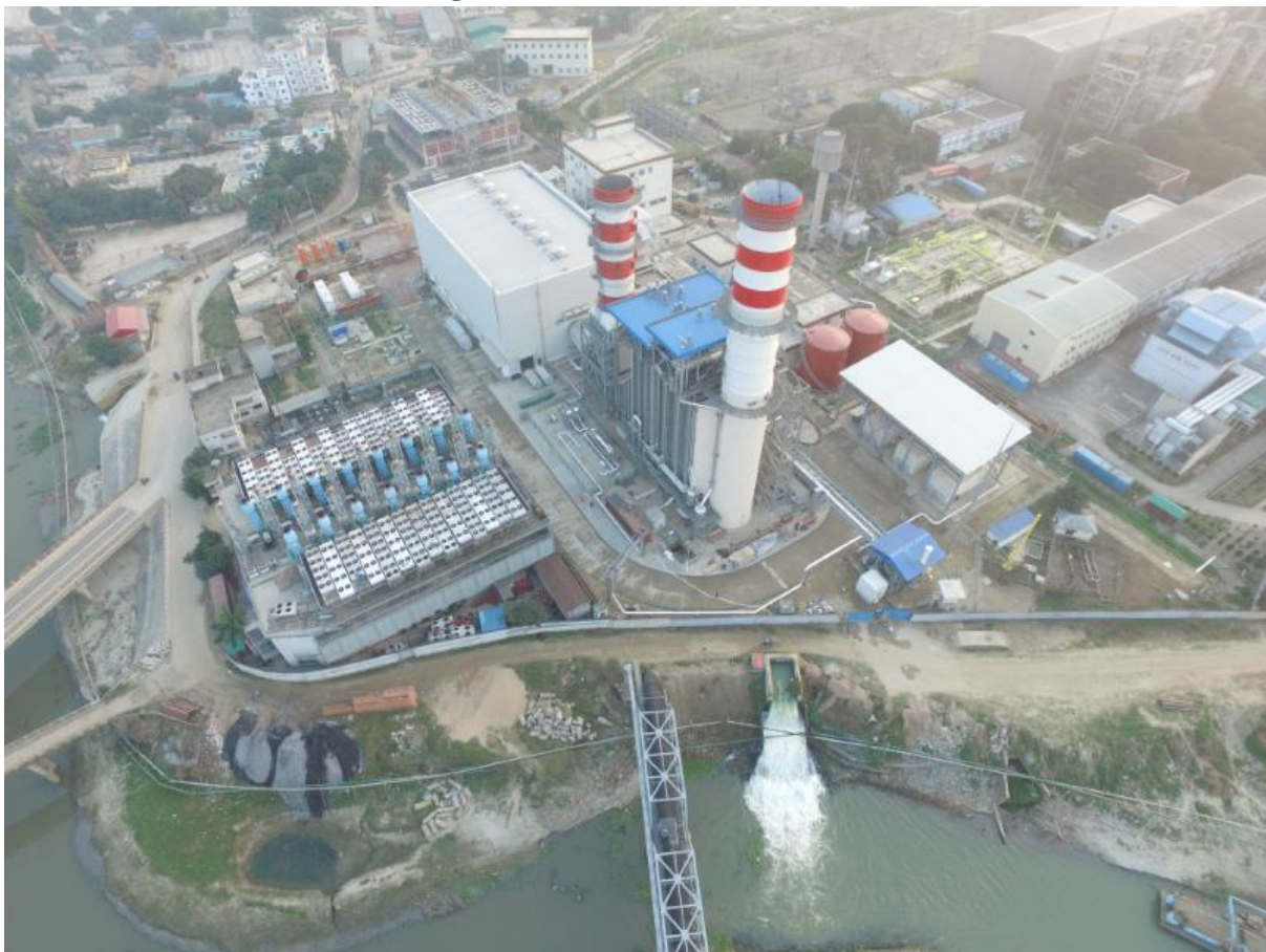
Figure 3: Latest Picture of the Project Site (Construction going on)
