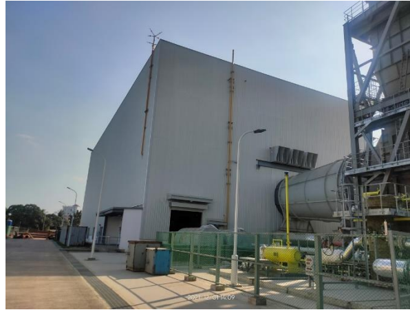
Fig.1.2.2: Construction of Turbine & Generator Hall
