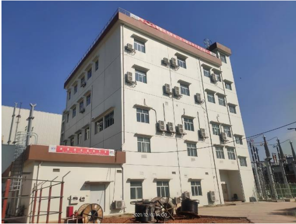
Fig. 1.2.1: Construction of Central Control Building (CCB)
