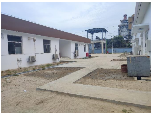
Fig. 1.2.7: Construction of watertreatment plant
