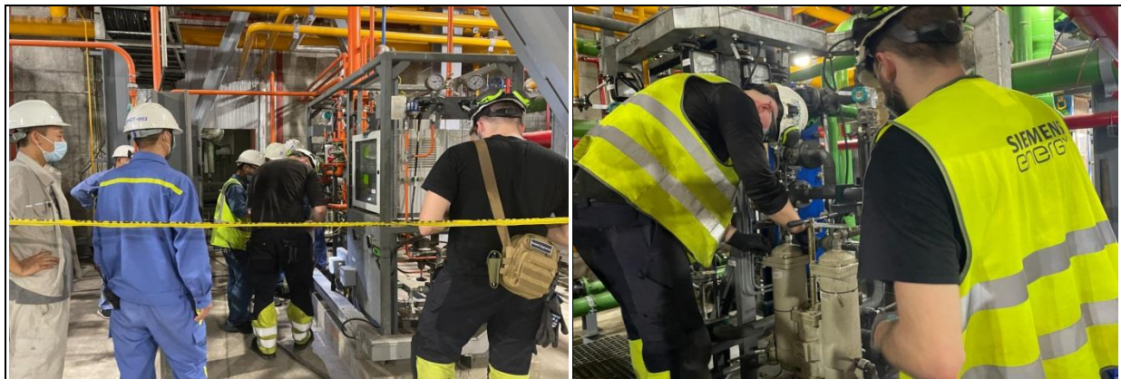
Figure 8: Use of Proper PPEs during Works
