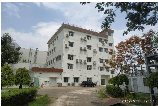
Fig. 1.2.1: Construction of Central Control Building (CCB)
