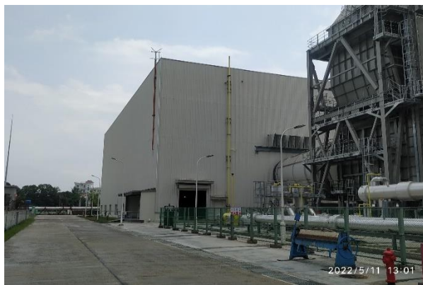
Fig.1.2.2: Construction of main building
