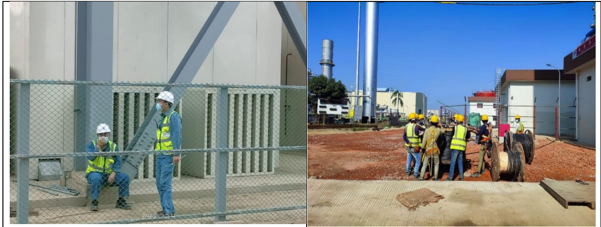
Figure 6: Use of Proper PPEs
