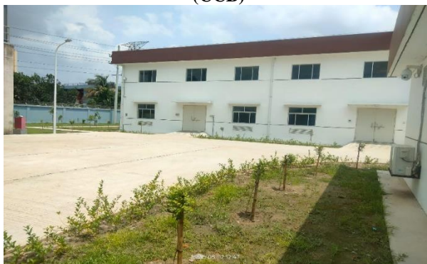
Fig. 1.2.4: Construction of chemical plant & Plantation at site
