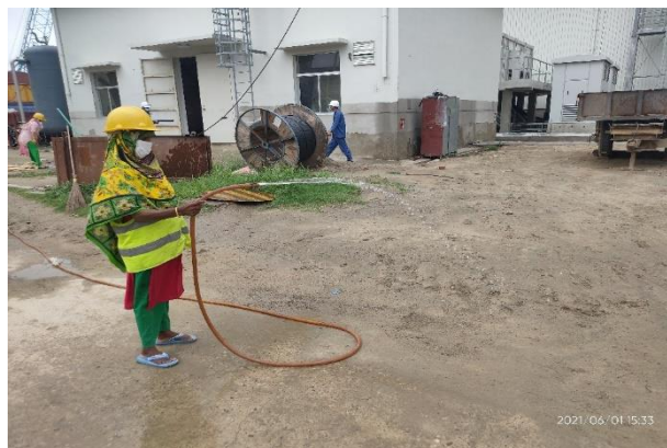
Figure 222: Water spraying for dust control.
