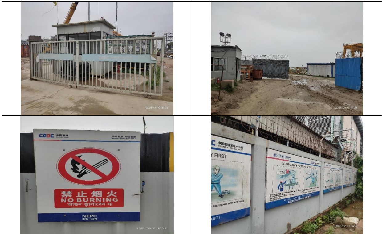
Figure 12: Site Security & Safety Instruction Board
