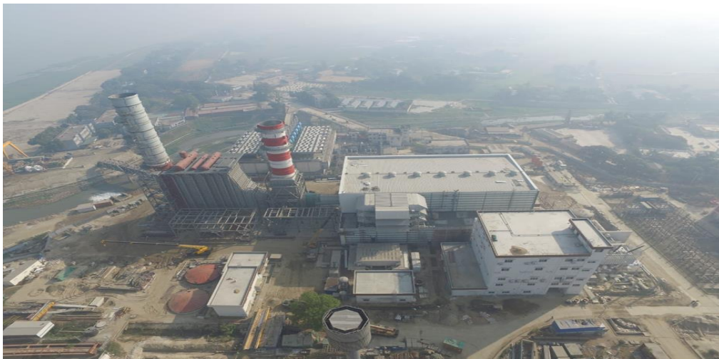
Figure 3: Latest Picture of the Project Site (Construction going on)
