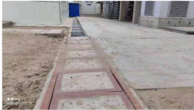
Figure 21: Cover slab on the top of drain
