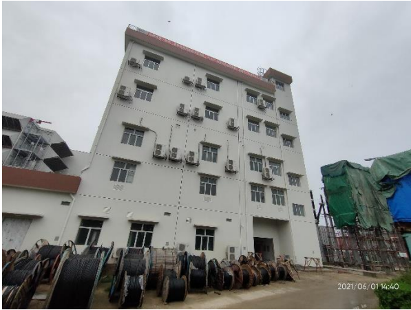
Construction of Central Control Building (CCB)
