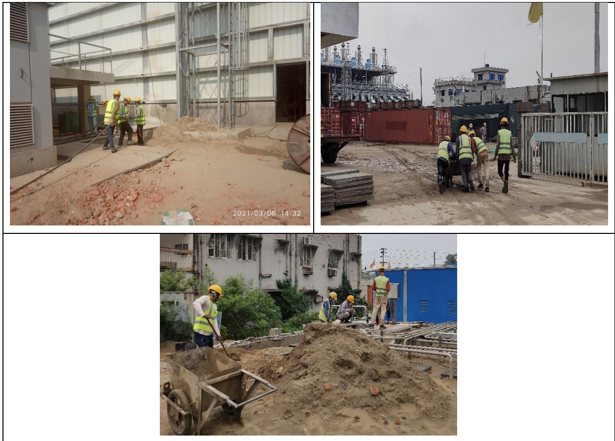
Figure 13: Use of Proper PPEs
