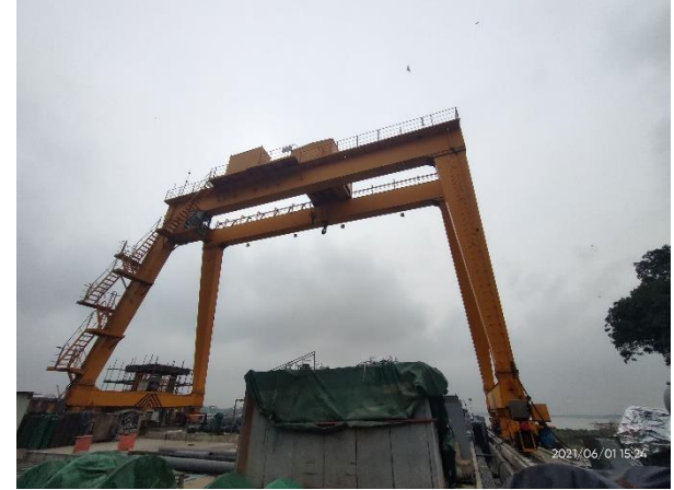
Water intake plant
