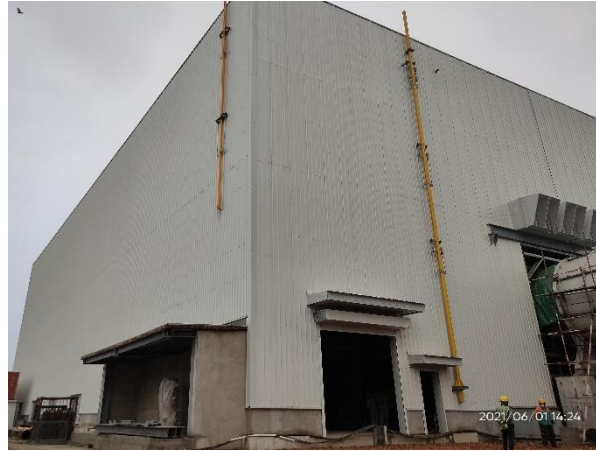
Construction of Turbine & Generator Hall
