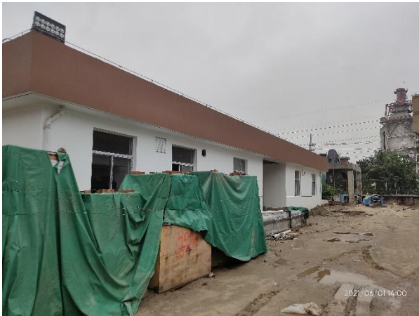
Construction of chemical plant
