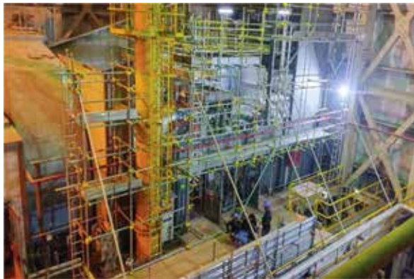
Scaffolding for dismantling GT Enclosure
