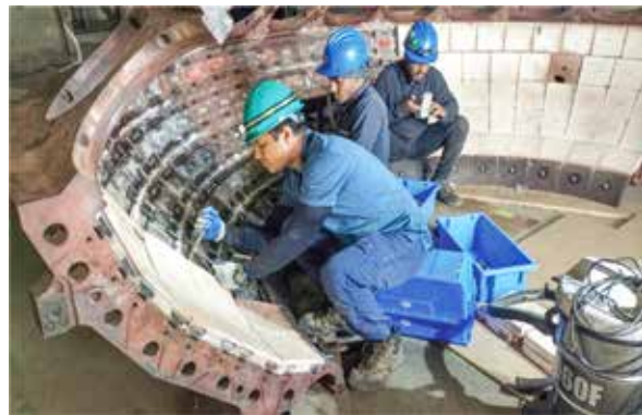
Combustion Chamber Tiles Removal
