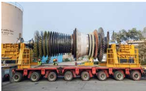
Rotor Transfer from North Turbine Hall to South Turbine Hall
