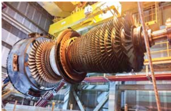
Rotor Lifting
