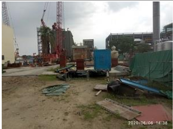
Fig: Construction of RMS Building
