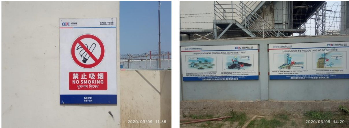
Figure-11: Sign boards and pictorial safety at the Project Site
