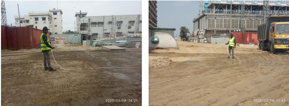
Figure -20: Water is spraying for dust control
