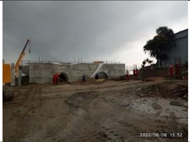
Fig: Construction of water intake plant
