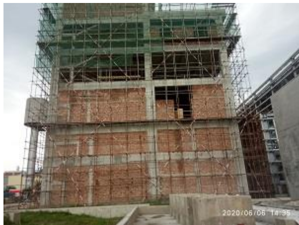
Fig: Construction of Central Control Building (CCB)
