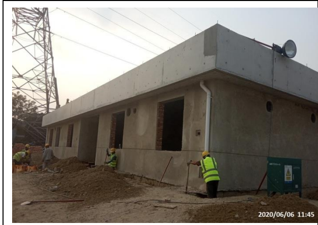
Fig: Construction of chemical plant
