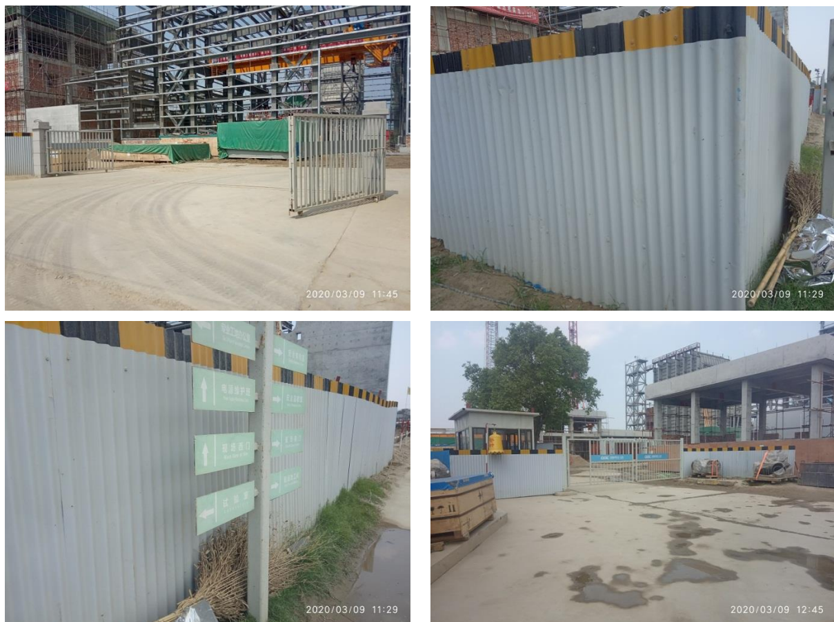
Figure-10: Present fencing conditions of the Project Site
