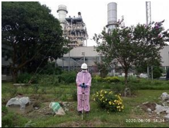
Fig.: Noise Quality Monitoring Location in front of Admin Building, APSCL
