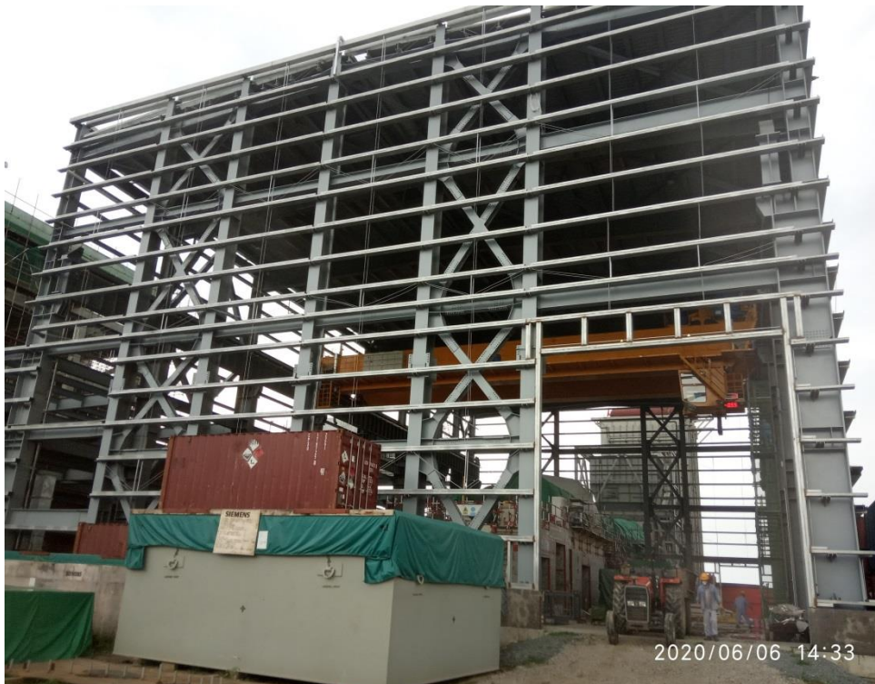
Fig: Photograph of Super structure construction of Main Building
