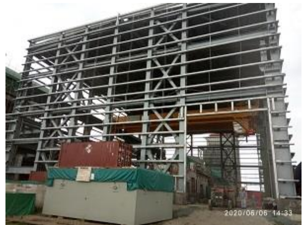
Fig: Construction of Main Building
