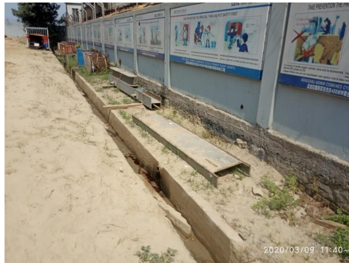
Figure-19: Existing outer drainage and rainy water reservoir
